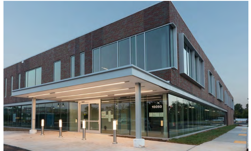
Kaiser Permanente Medical Office Building Haymarket, Virginia, Courtesy of RW Murray Co.
