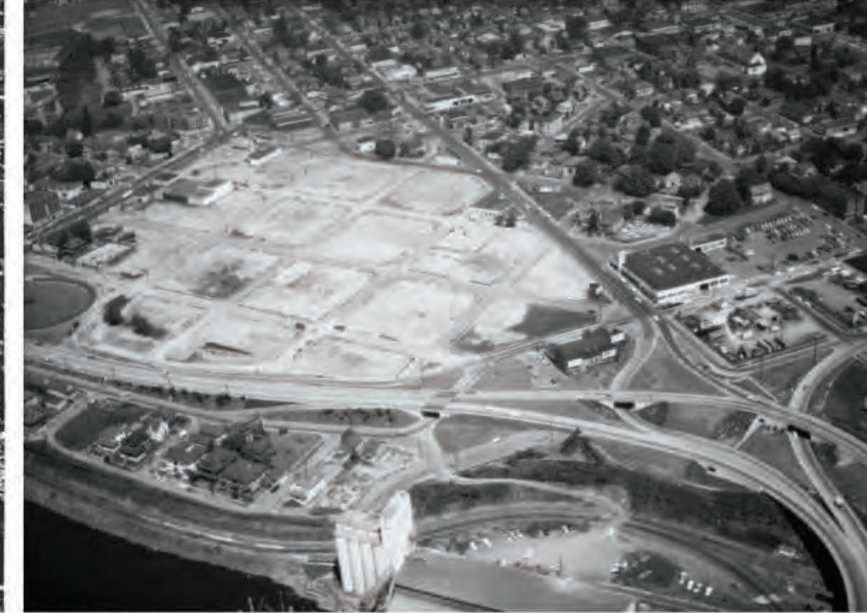
1958 SITE CLEARED FOR MEMORIAL COLISEUM
