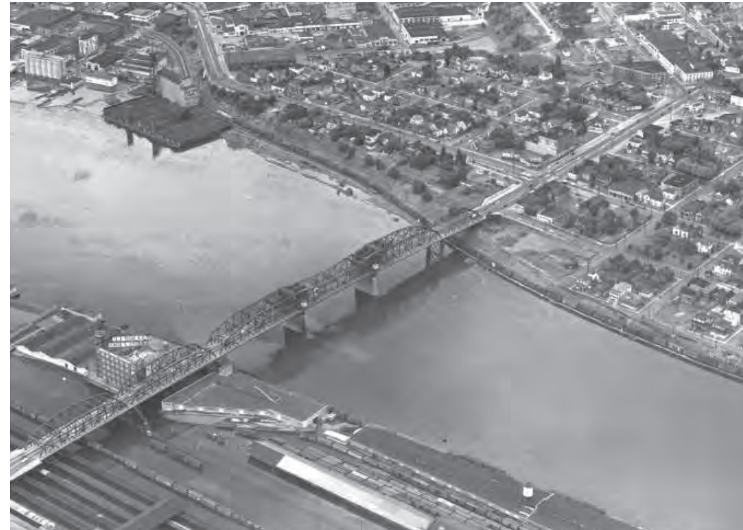
1948 Broadway Bridge during the Vanport Flood
