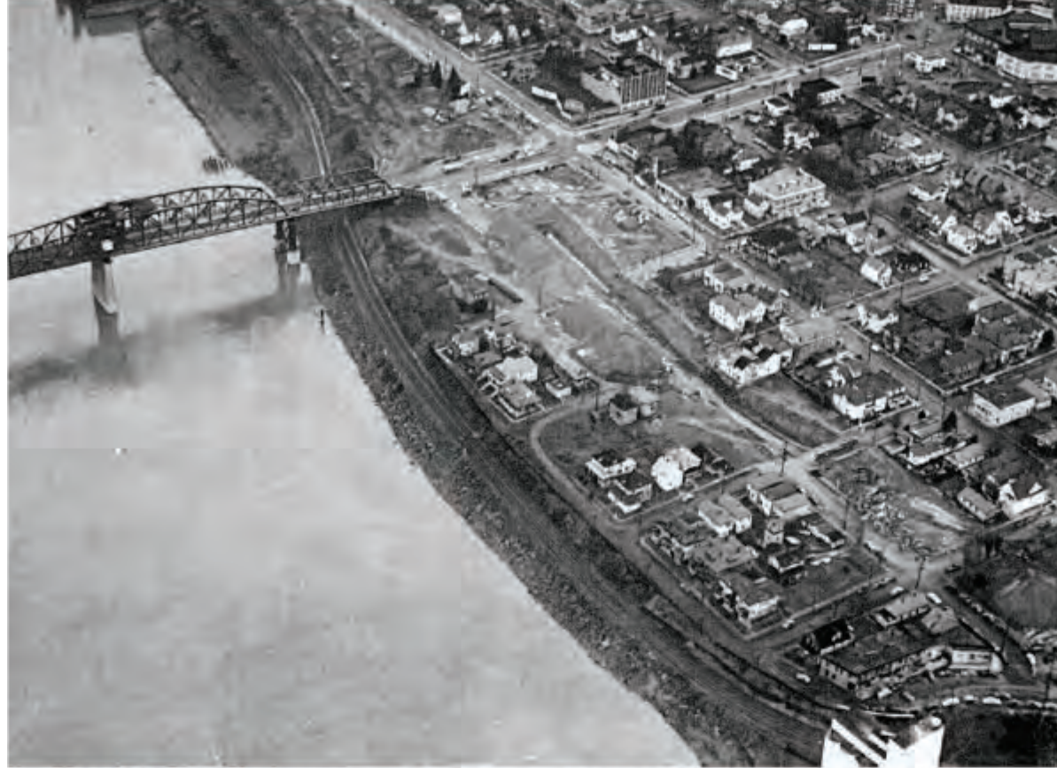
1949 CONSTRUCTION BEGINS ON INTERSTATE AVE
