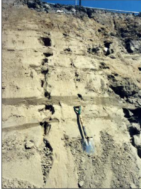
Figure 1-3. Fine-grained Bretz/Missoula flood deposits exposed in the foundation excavation of the Oregon Convention Center. Dark bands are damp paleosols mark the tops of some rhythmites.
