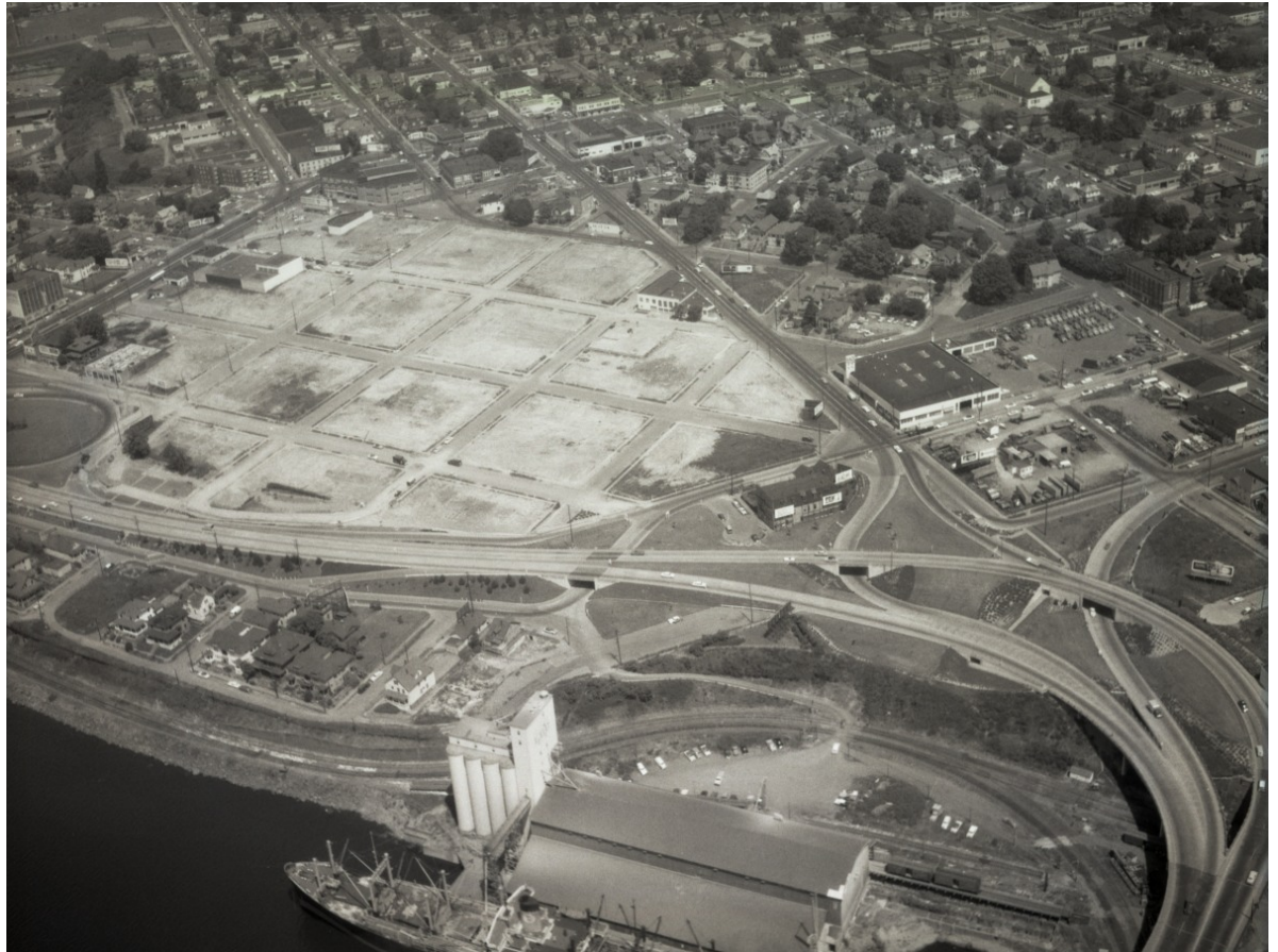
Figure 26. Location of the Memorial Coliseum – During Construction (ca. 1955). Photo shows houses and streets from Figure 25 demolished. View is to the northeast.
