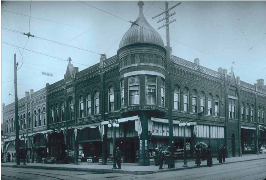
Figure 19. Hill Block Building, 1910. Located on the NW corner of N Russell and N Williams.
