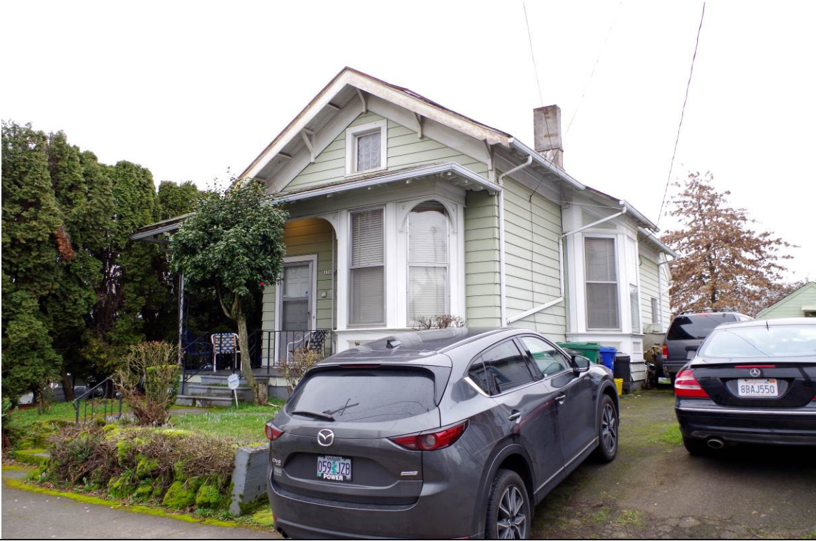
View: 1745 NE 1st Avenue, East façade, viewing southwest
