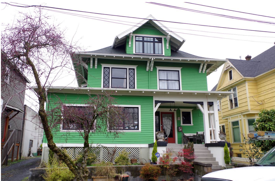
View: 23 NE San Rafael Street, facing north
