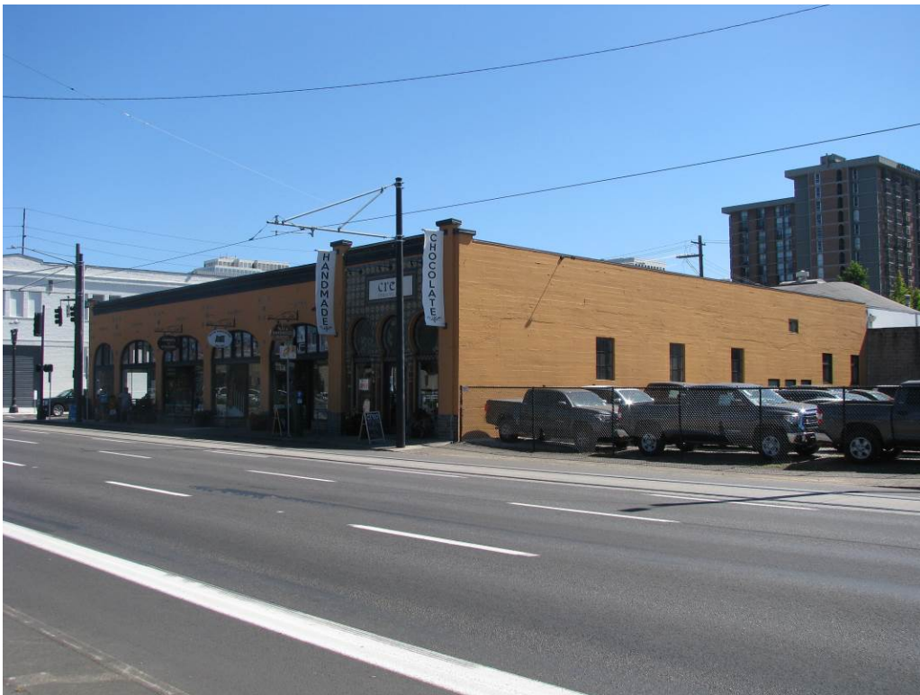
View: West and north elevations, viewing southwest
