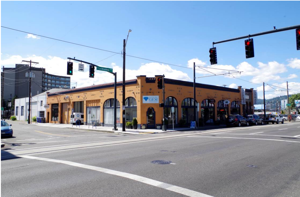
W. E. Field Tile Co. Building viewing southwest
