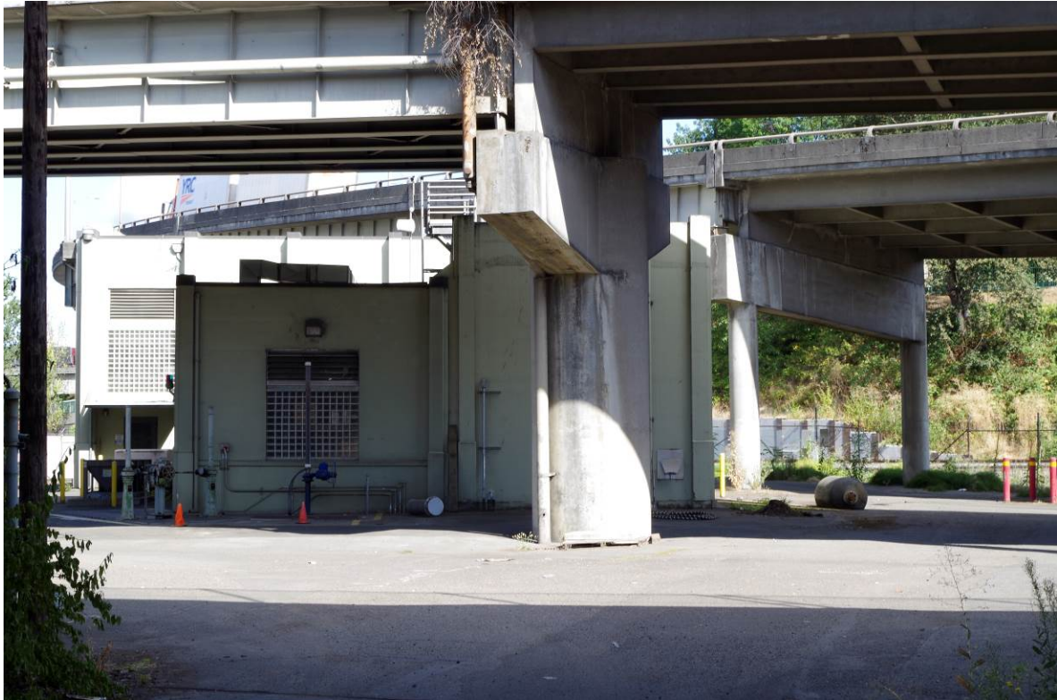
View: South elevation, viewing northwest
