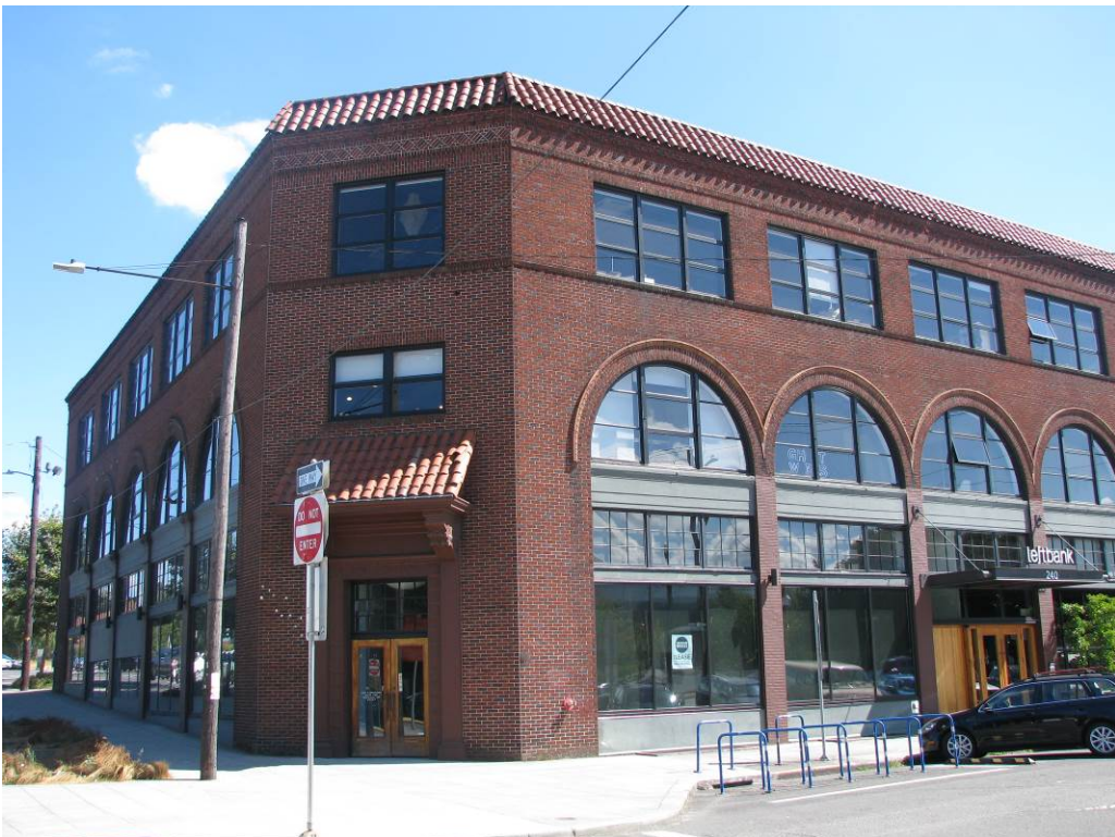
View: Northwest elevation, viewing northeast
