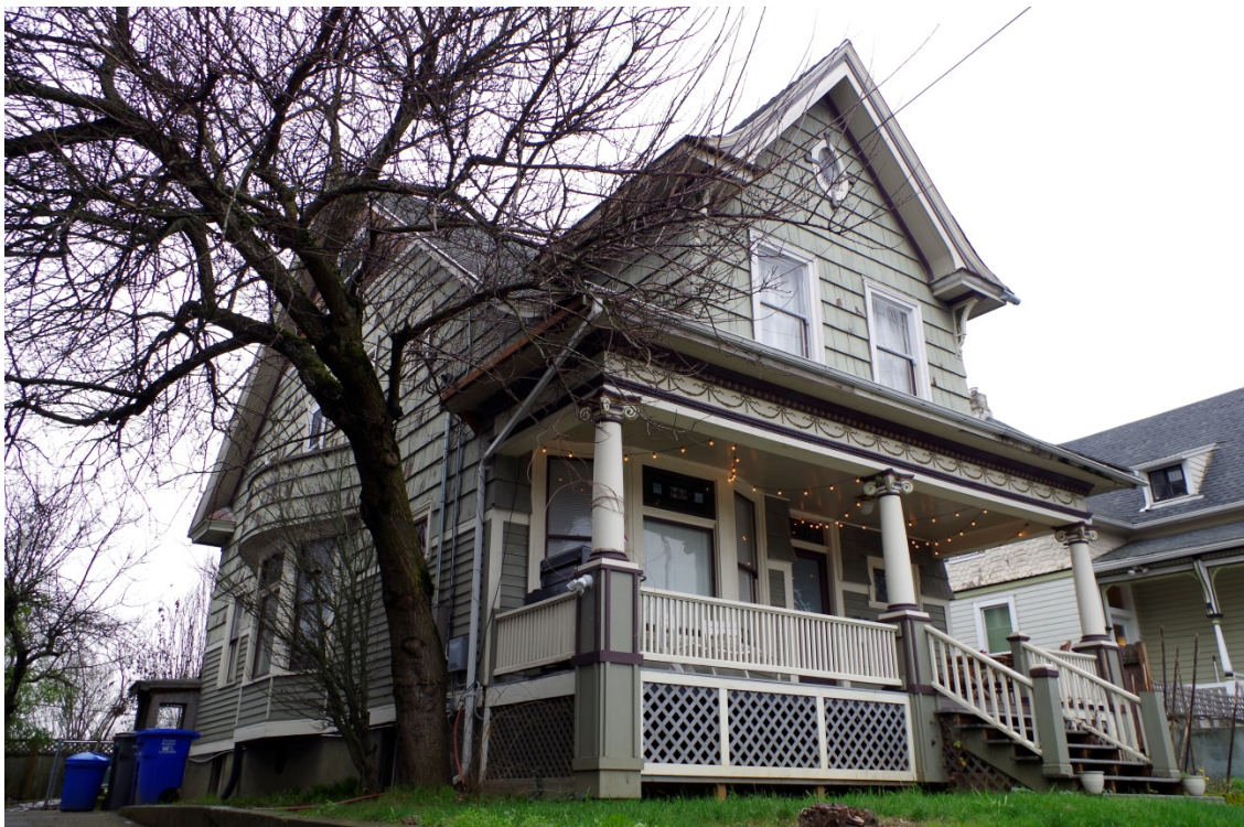
View: South elevation, viewing northwest
