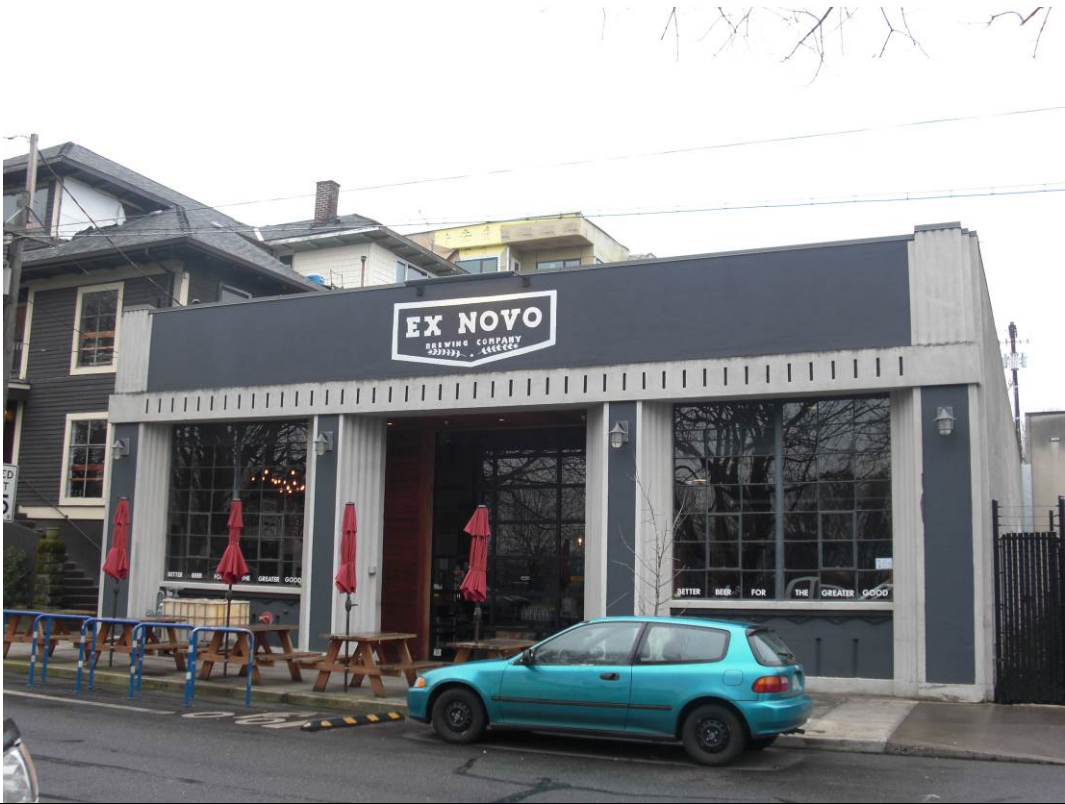
View: West façade, viewing northeast
