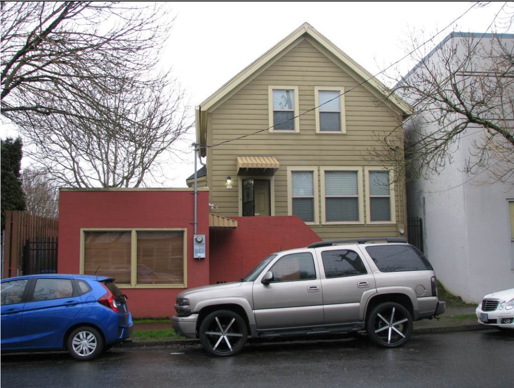
View: South façade, viewing north
