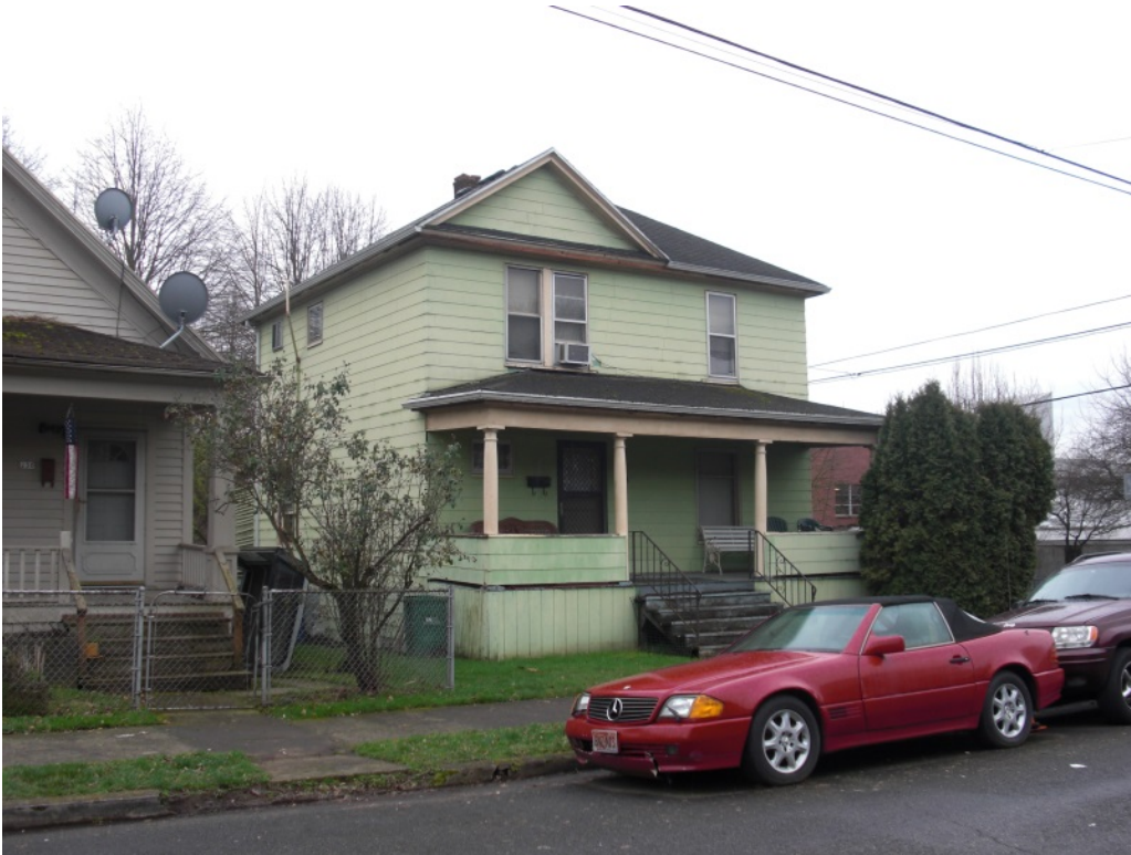
View: 236 N Page Street, North (façade) and East elevations, viewing southwest
