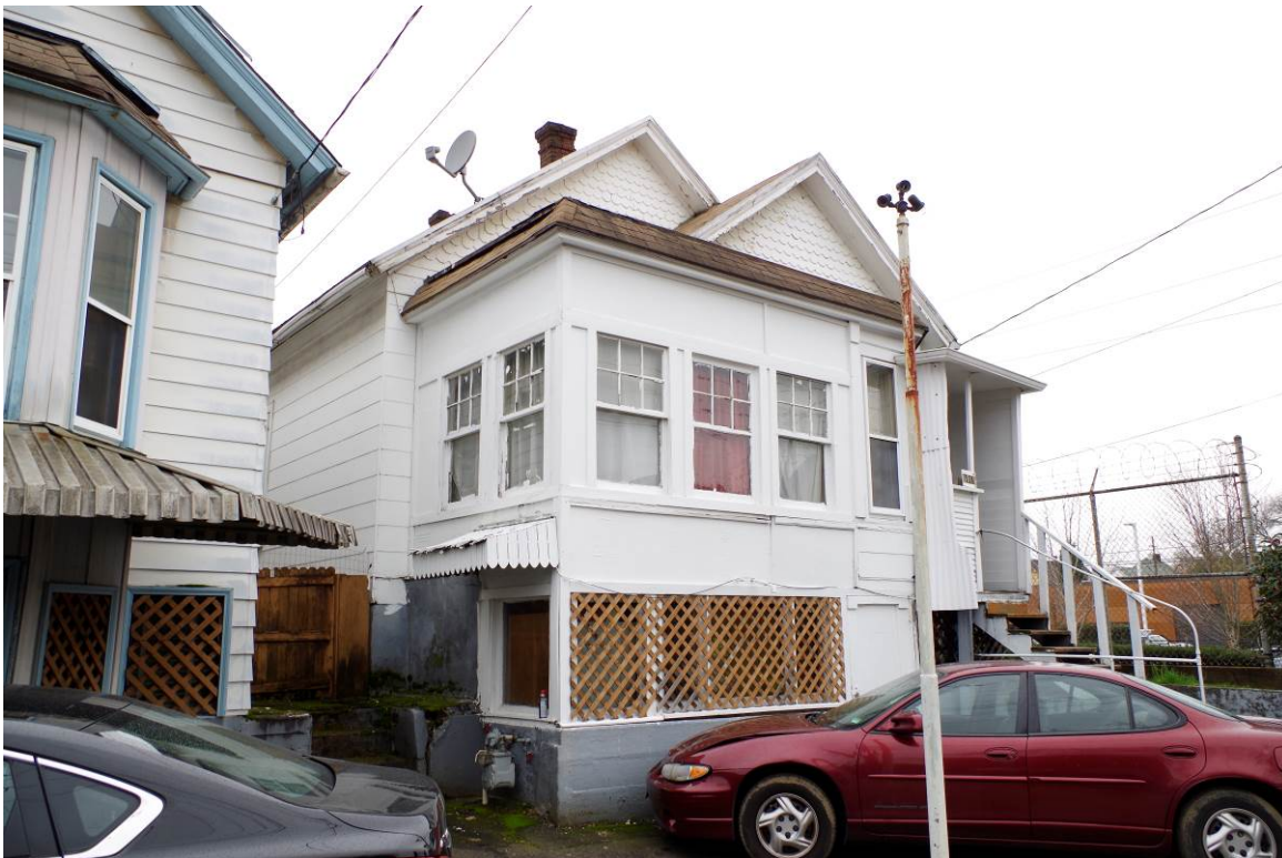
View: 1811 NE 1st Avenue, South elevation and East façade, viewing northwest
