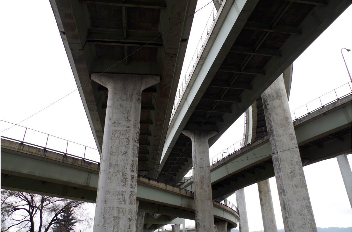
View: Fremont Bridge, viewing southwest
