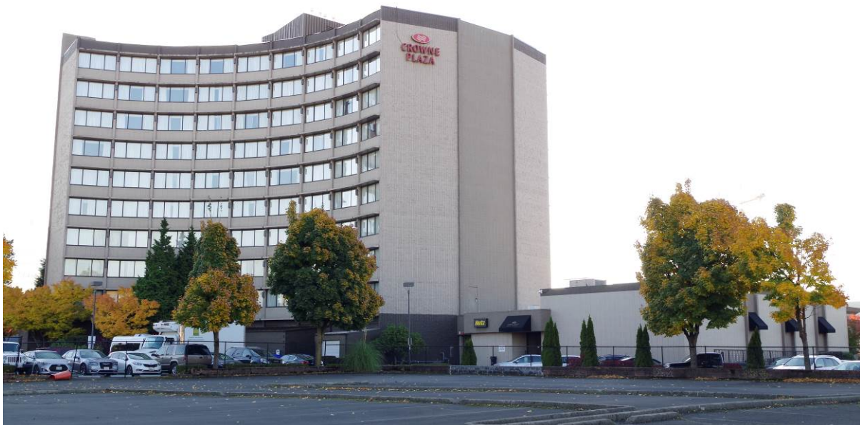
View: West elevation, viewing southeast
