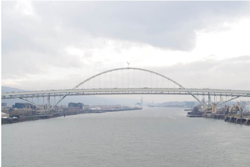
Fremont Bridge viewing northwest
