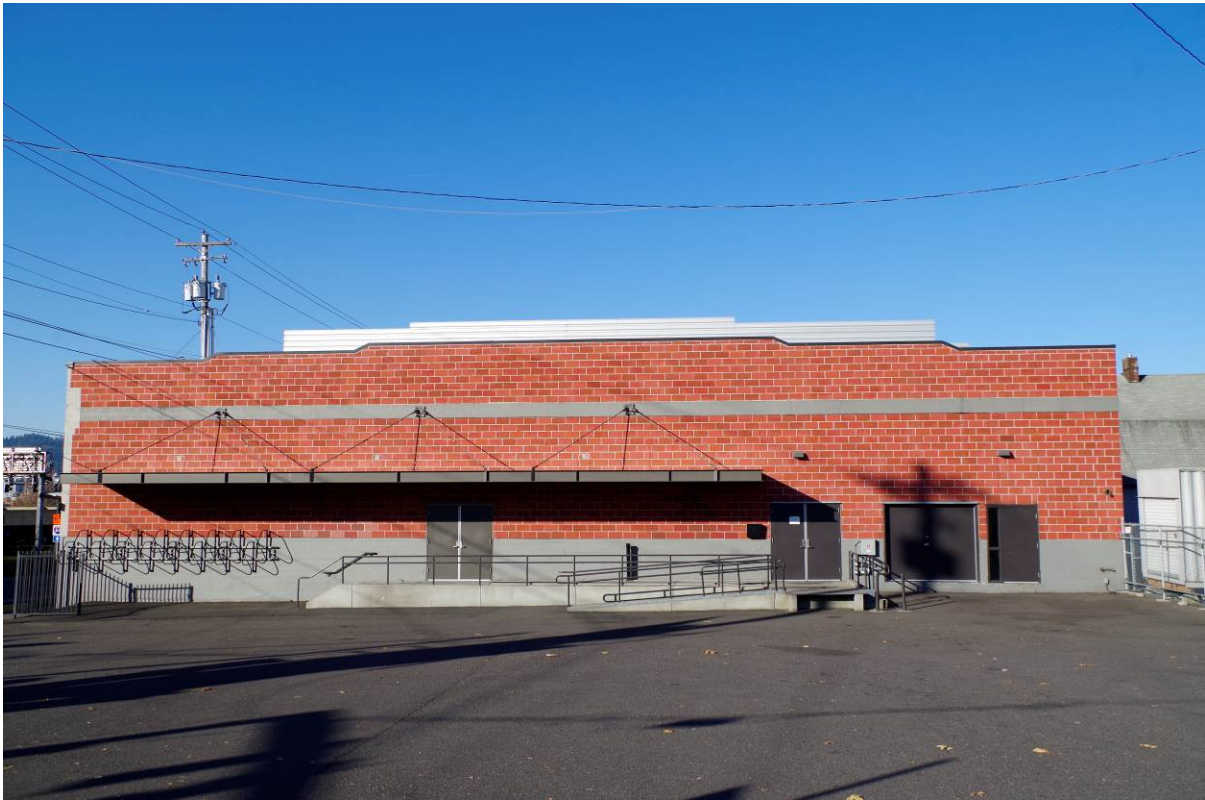
View: East elevation, viewing northwest
