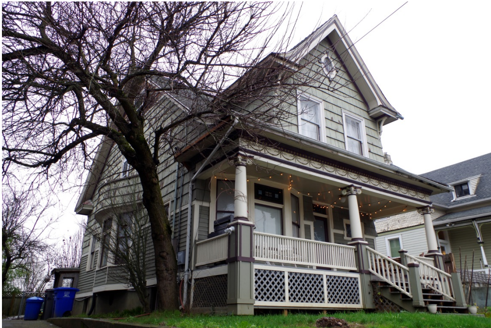
Charles E. and Emma E. Holzer House viewing northwest
