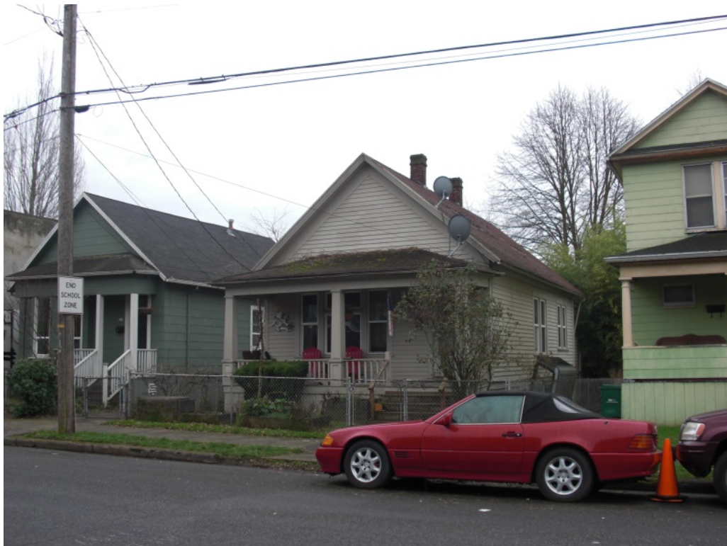
View: 230 N Page Street, North (façade) and West elevations, viewing southeast
