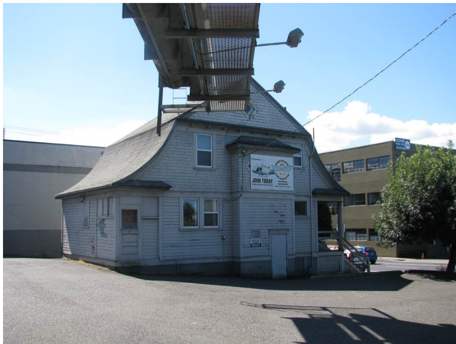
View: North and east elevations, looking southwest.
