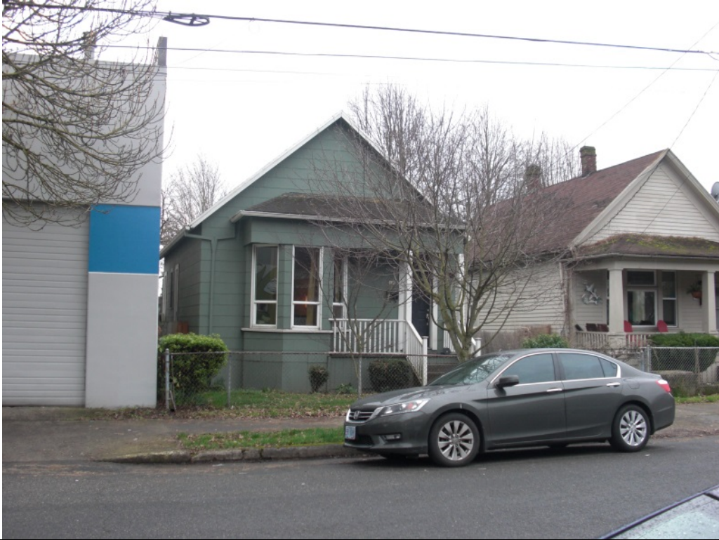
View: 226 N Page Street, North (façade) elevation, viewing south
