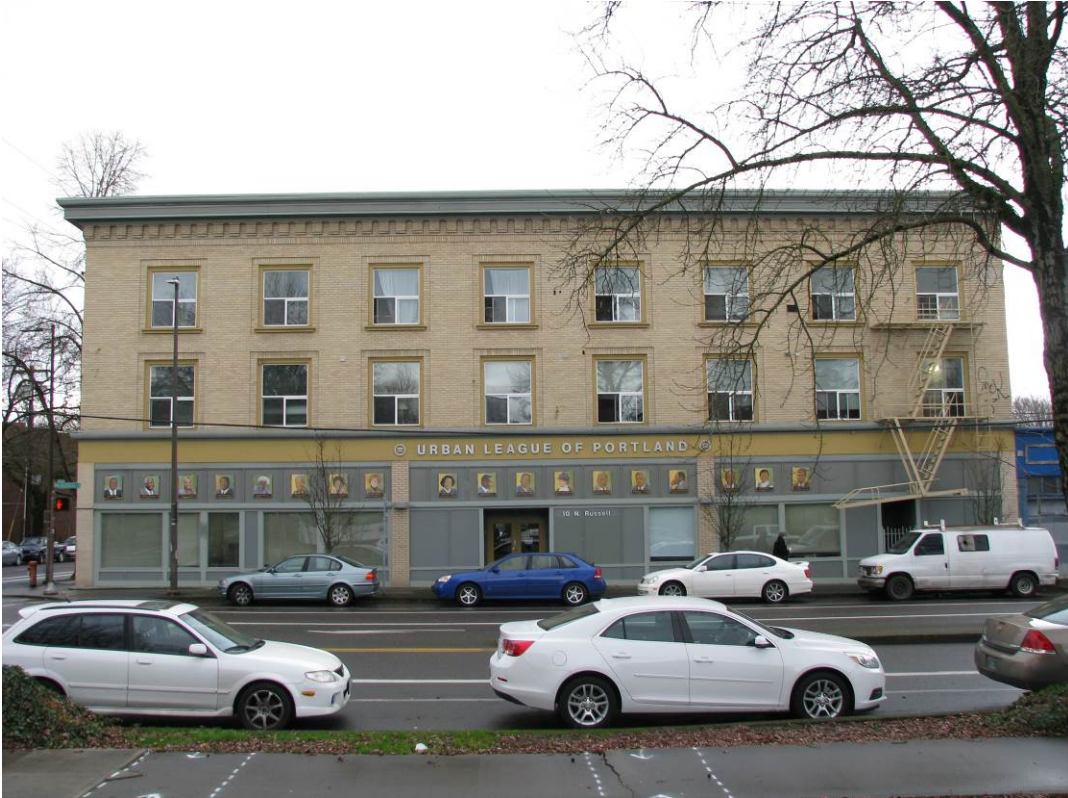
View: North elevation, viewing south
