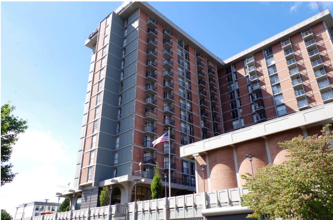
View: North and east elevations, viewing southwest
