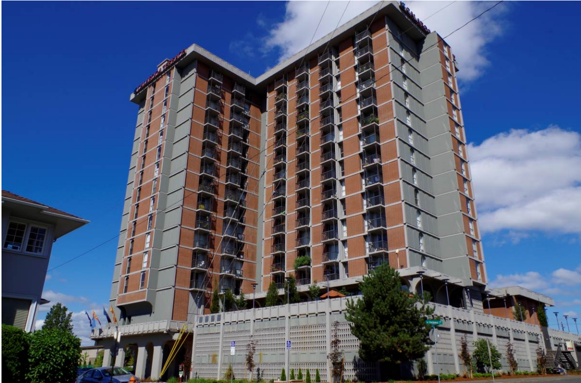
View: South and east elevations, viewing northwest
