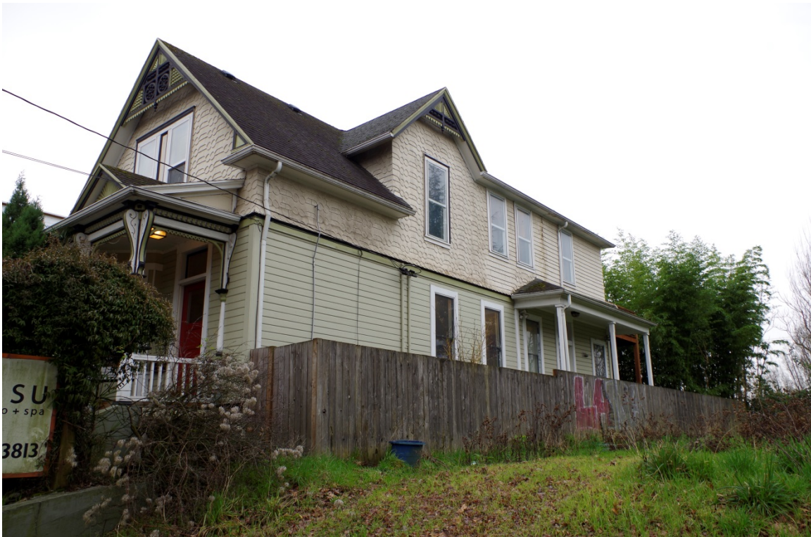
View: North elevation, viewing southwest
