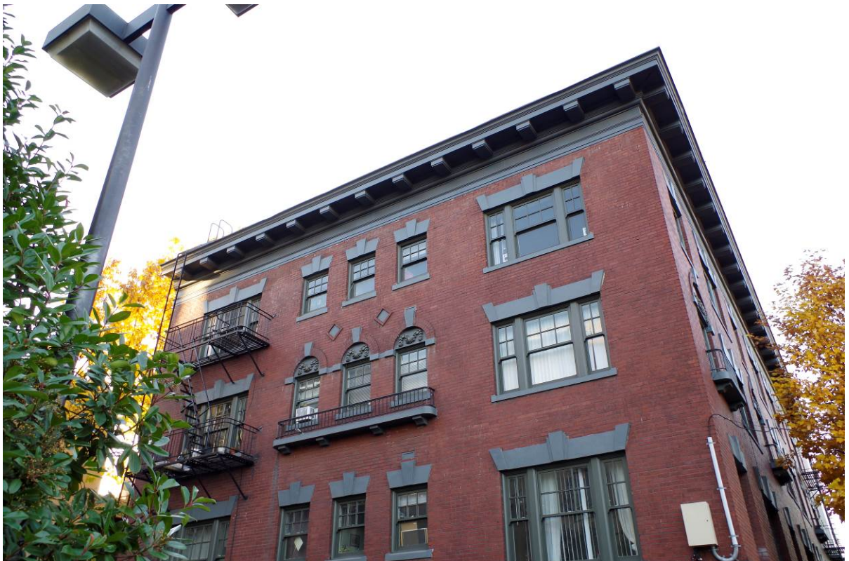
View: North elevation, viewing southeast
