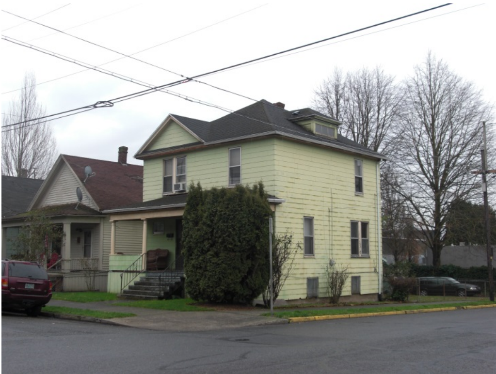
View: 236 N Page Street, North (façade) and West elevations, viewing southwest
