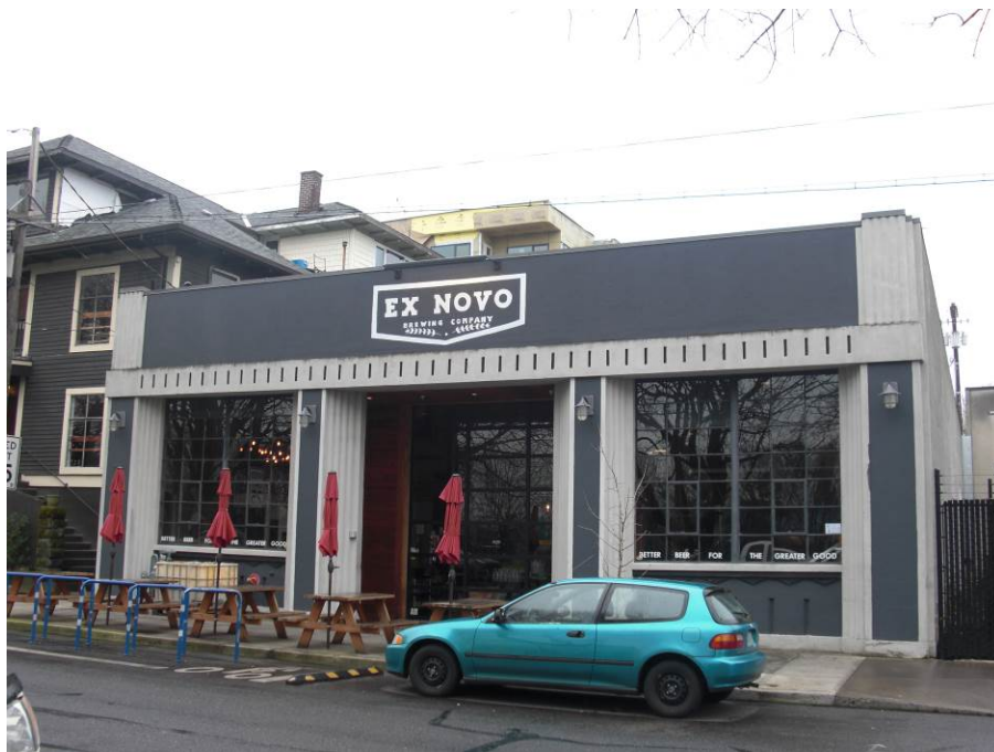
Contractors Warehouse viewing northeast
