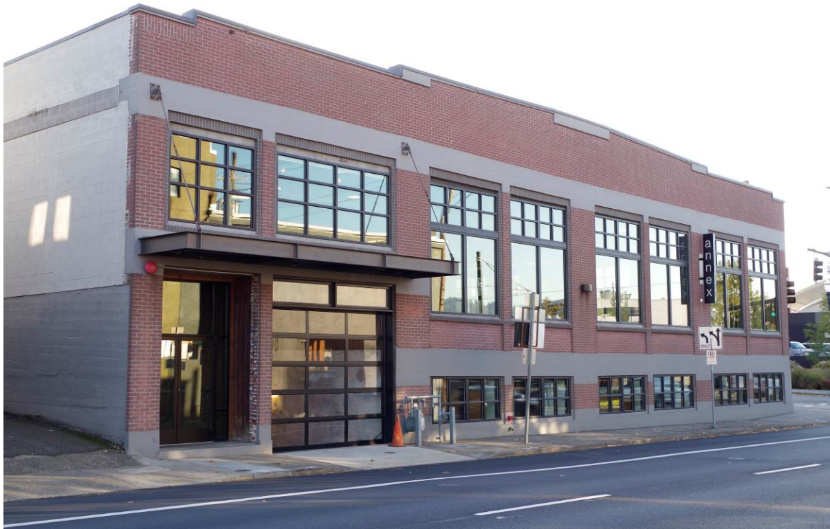
View: West elevation, viewing southeast
