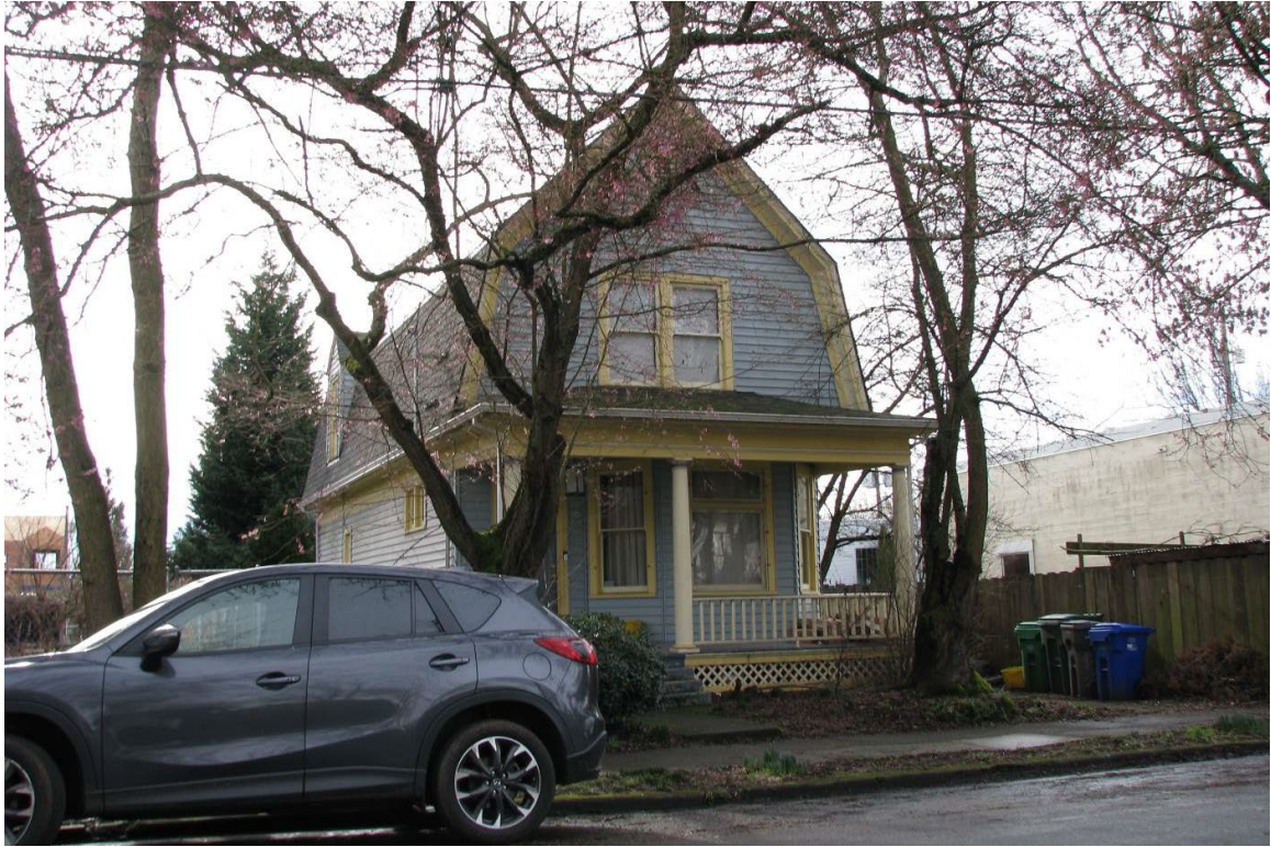
View: 20 NE Thompson Street, facing southwest
