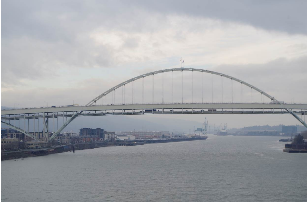
View: Fremont Bridge, viewing northwest
