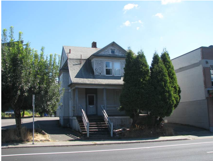
View of Daskalos House viewing east
