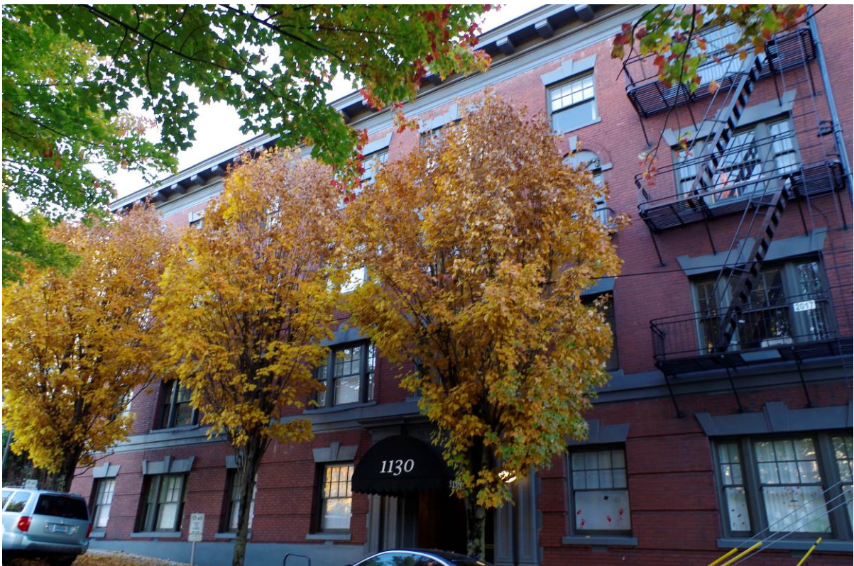
View: West façade, viewing northeast
