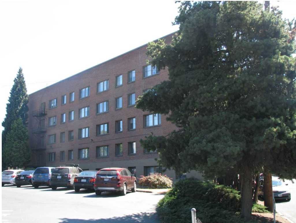
View: North elevation, viewing southeast
