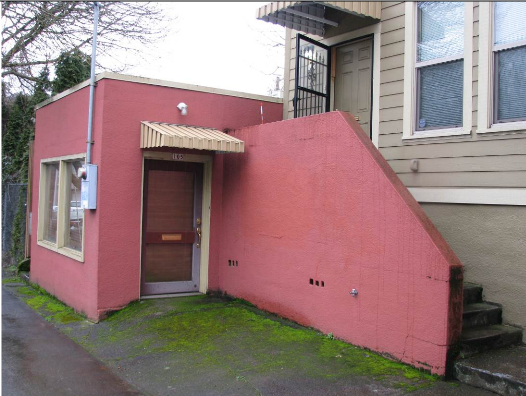
View: Barber Shop Addition, viewing northwest
