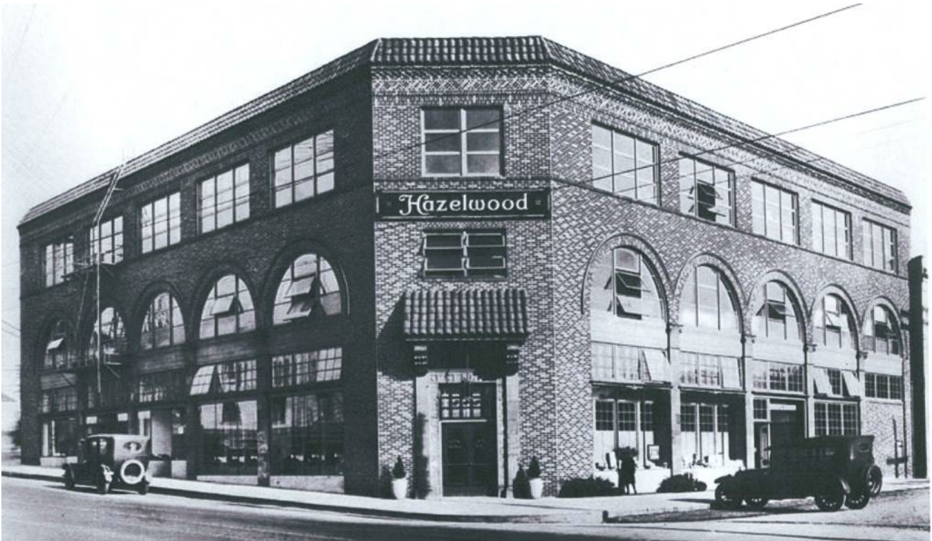
View: Historical aerial view, looking southeast, 1930s. See Agee, Joanna. (n.d.). "The Hazelwood." National Register Preliminary Eligibility Evaluation Form for Historic Resources. Salem, OR: Oregon State Historic Preservation Office.
