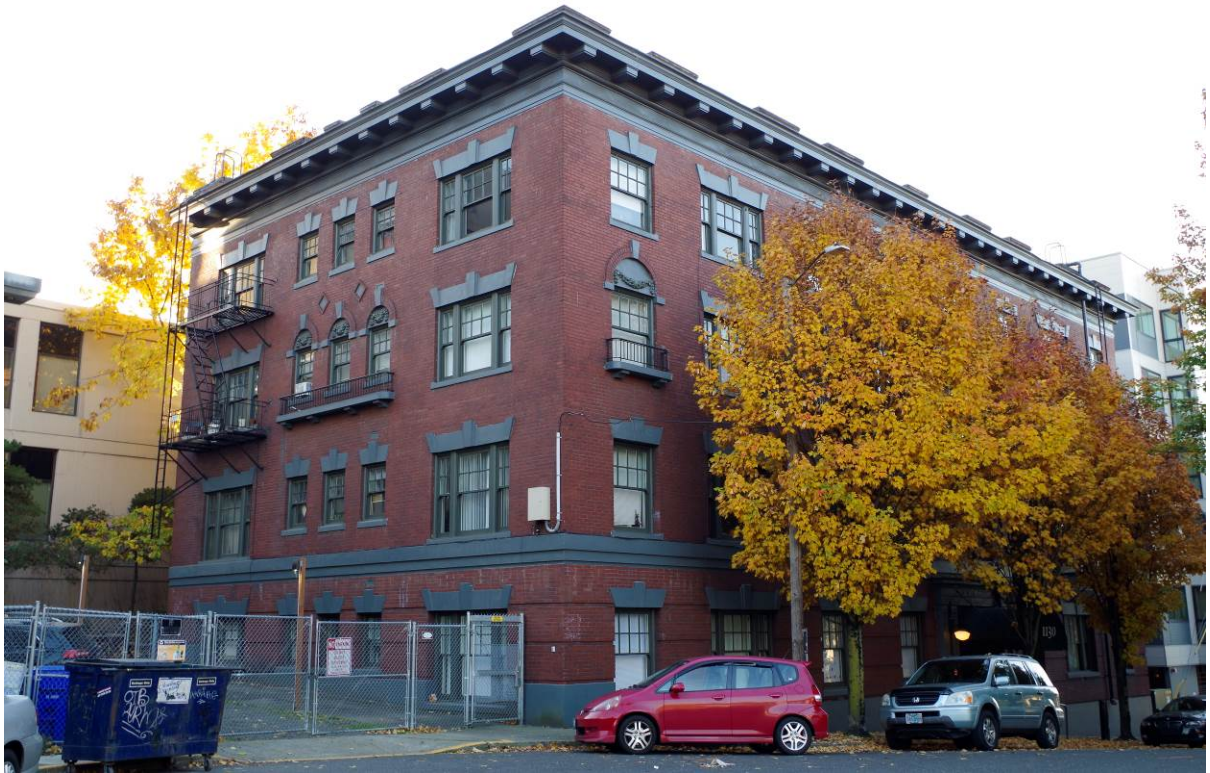
View: West façade, viewing southeast
