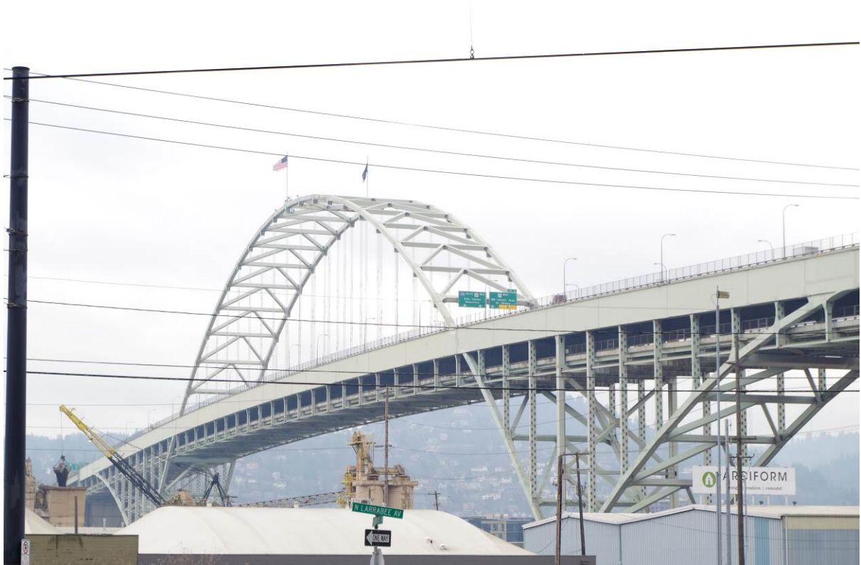
View: Fremont Bridge, viewing west
