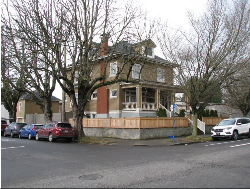
View: East façade, viewing northwest
