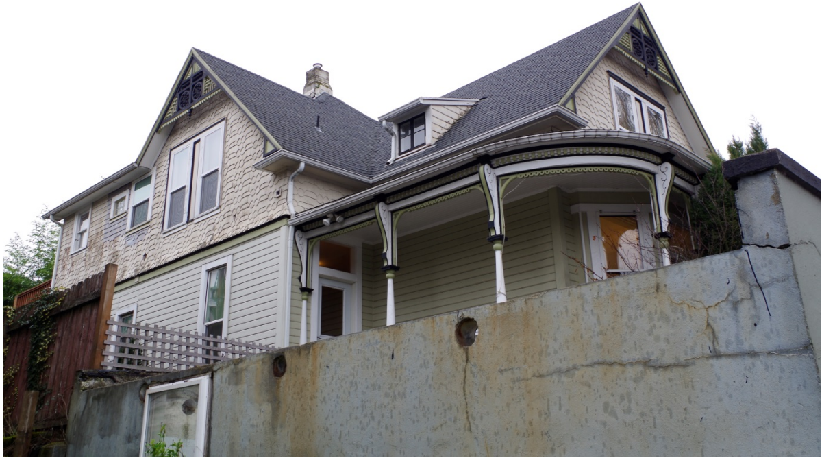
View: South elevation, viewing northwest
