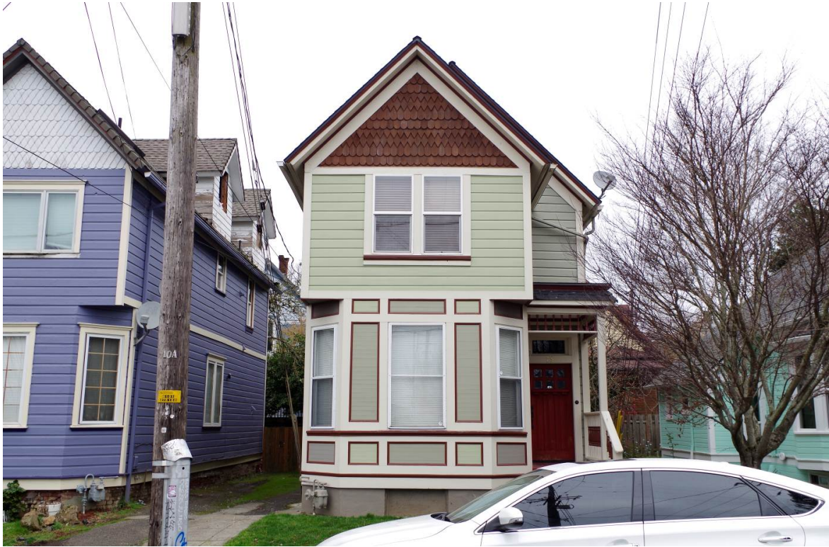
View: 73 NE Hancock Street, facing north
