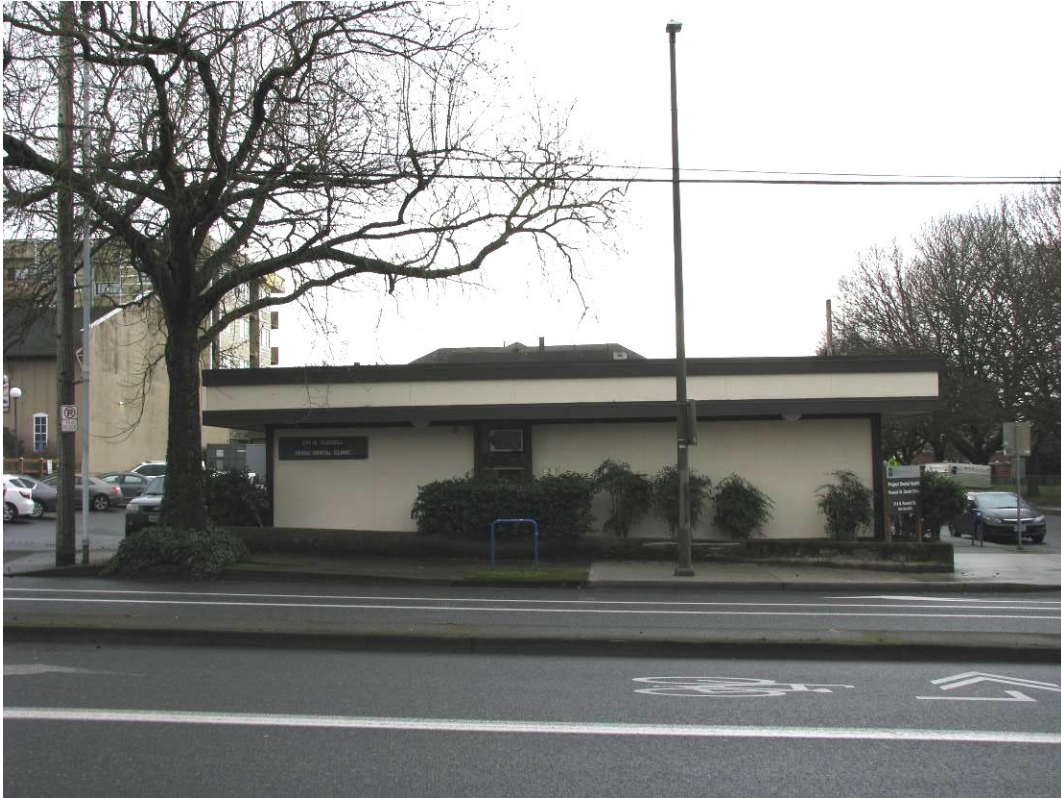
View: North elevation, viewing south
