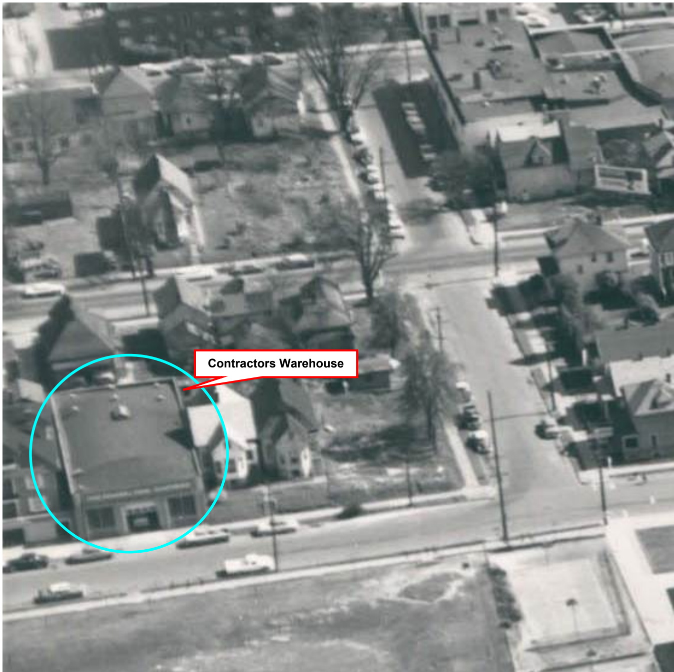
View: Historic view, viewing southeast, 1962. City of Portland Archives. See https://vintageportland.files.wordpress.com/2012/06/a2005-001-183-eastbank-freeway-with-broadway-weidler-couplet-1962.jpg
