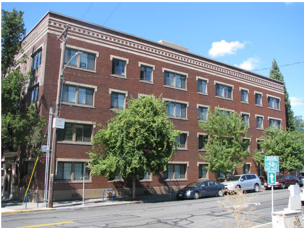
View: East elevation, viewing northwest
