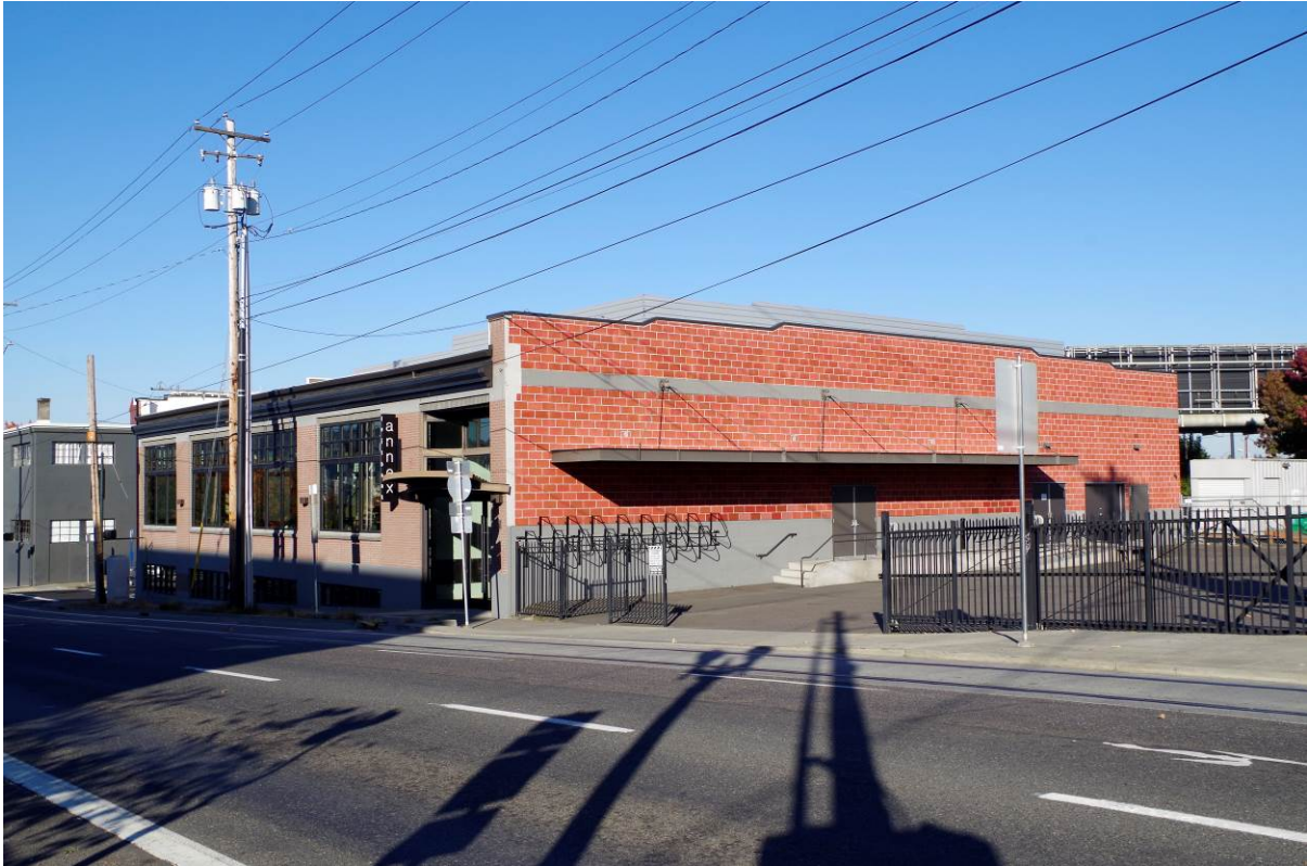
View: South elevation, viewing northwest
