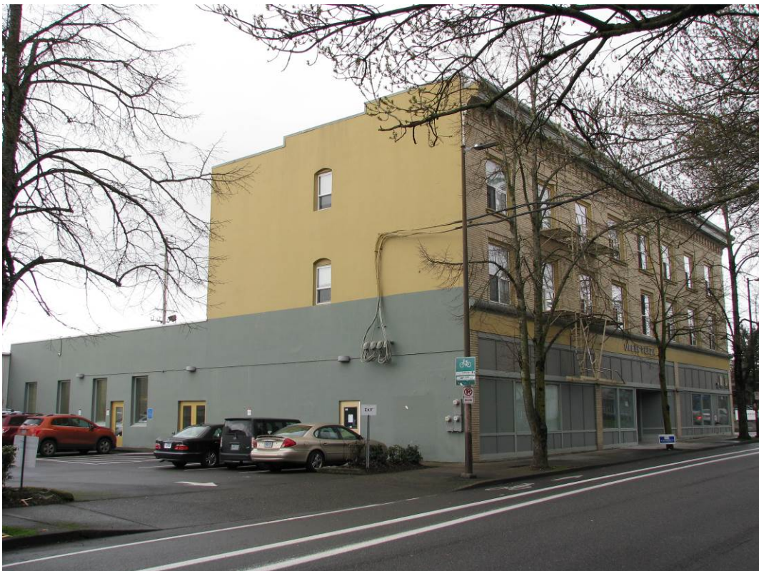
View: East and south elevations, viewing northwest
