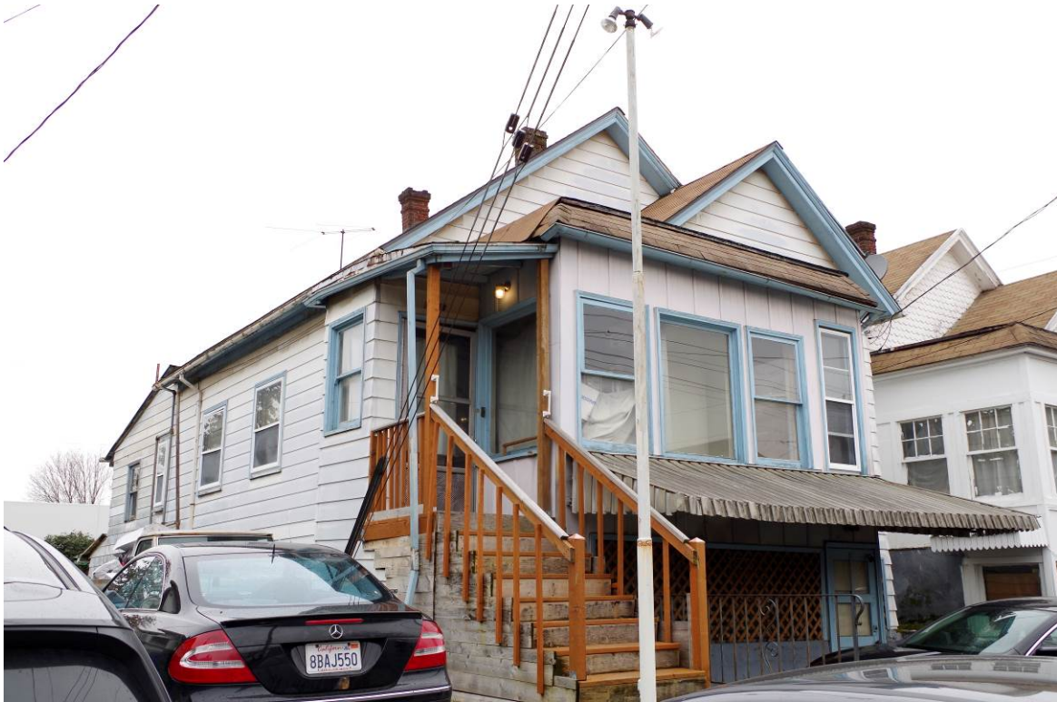
View: 1803 NE 1st Avenue, South elevation and East façade, viewing northwest
