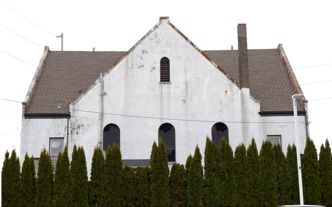
View: South elevation, viewing north
