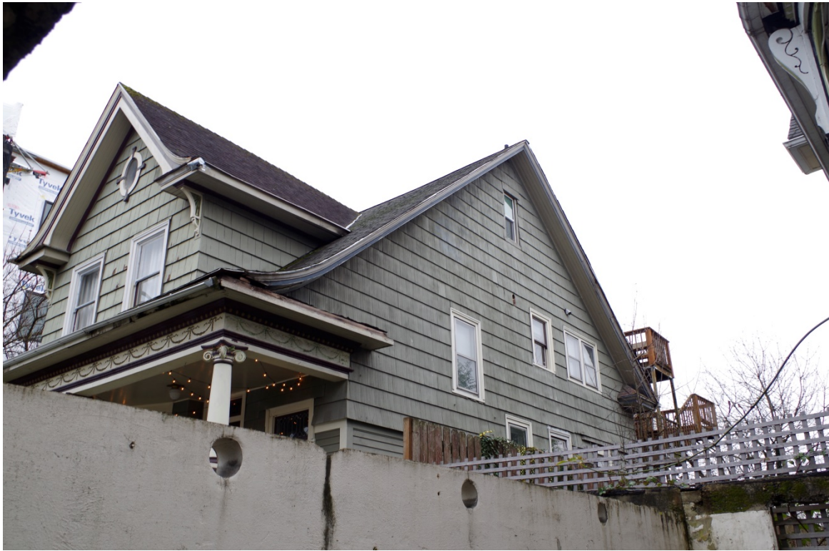
View: North elevation, viewing southwest
