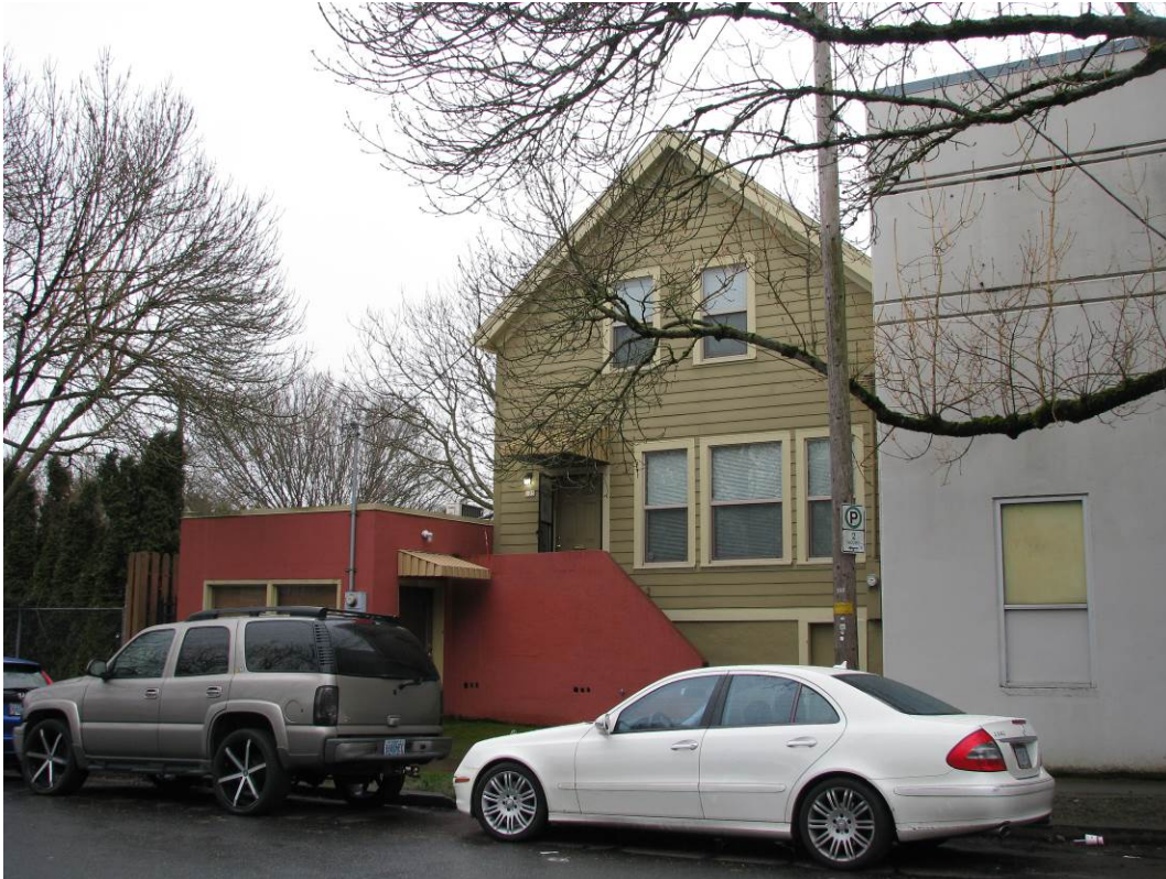
View: South façade, viewing northwest
