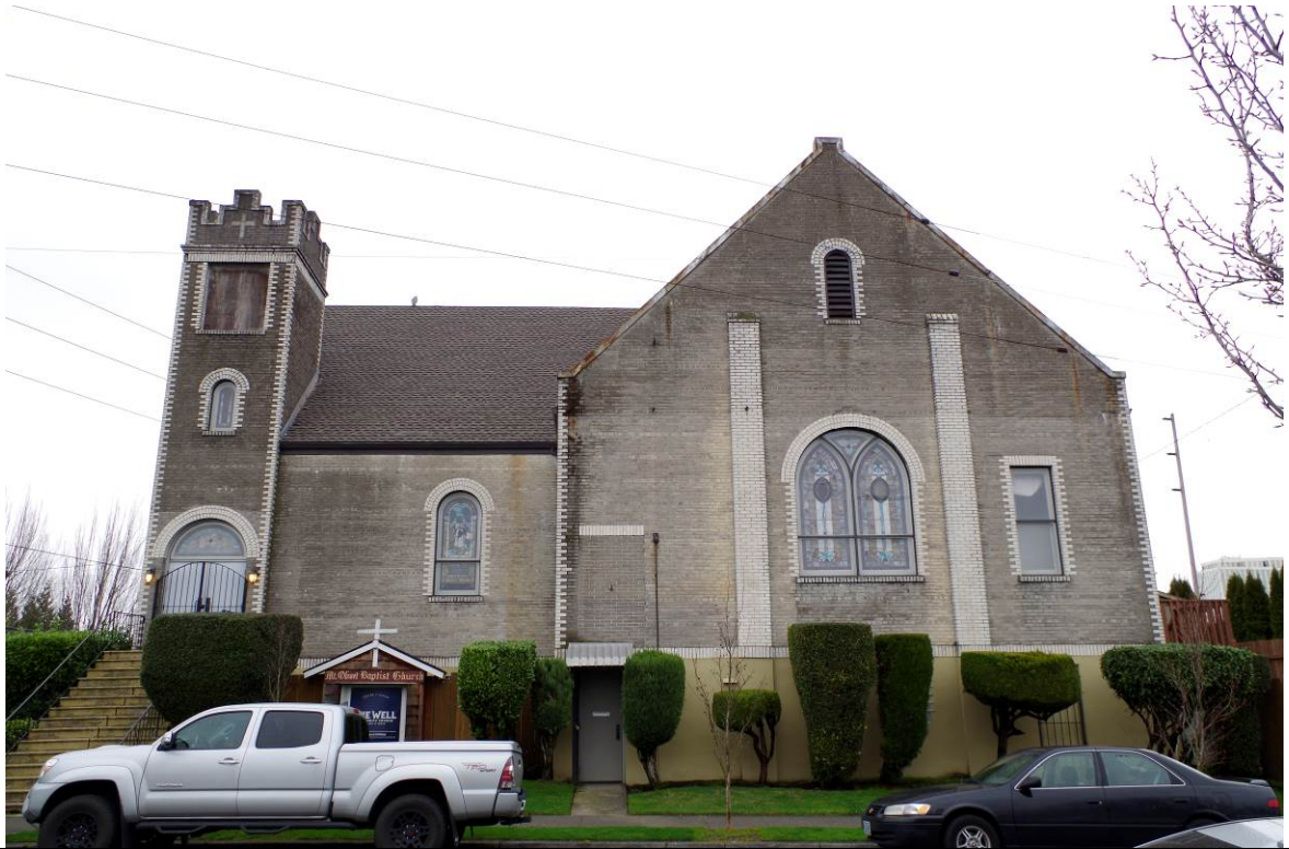
View: West elevation, viewing east
