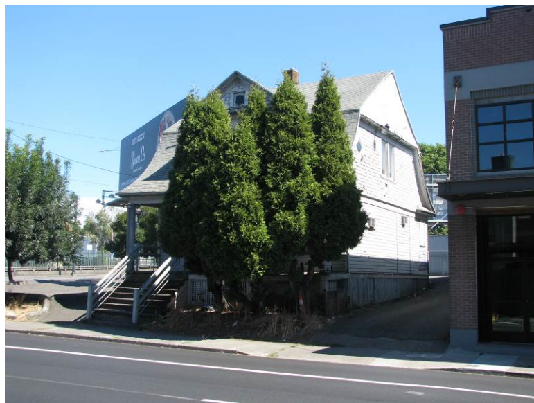
View: West and south elevations, looking northeast.
