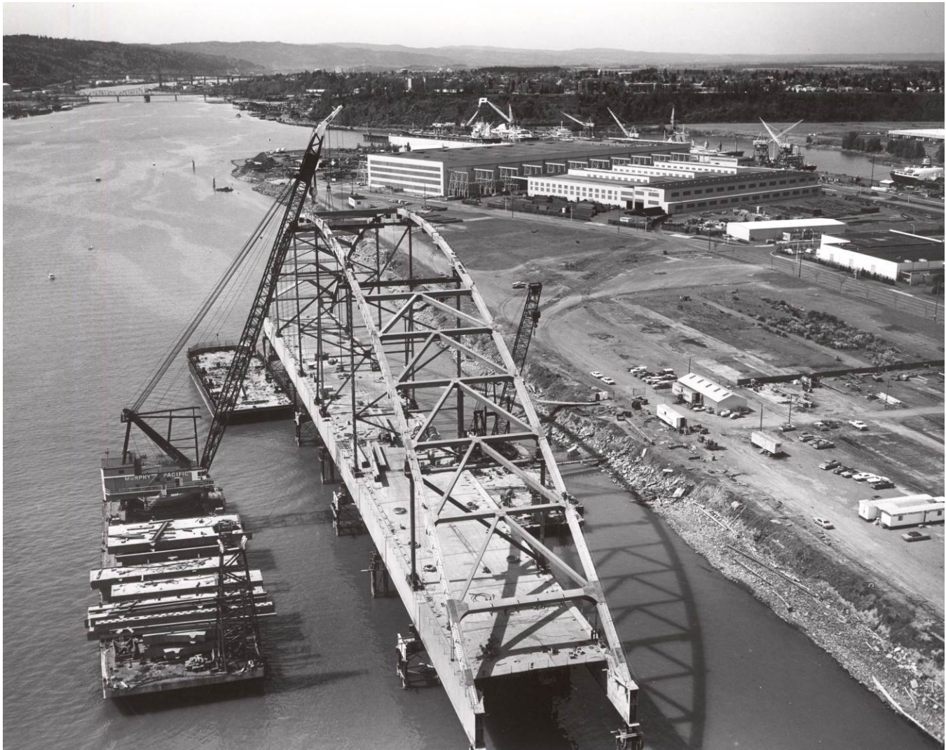
View: Historic view, viewing northeast, 1972. City of Portland Archives. See https://vintageportland.files.wordpress.com/2010/10/a1999-004-917-fremont-bridge-center-span-construction-swan-island-1972.jpg
