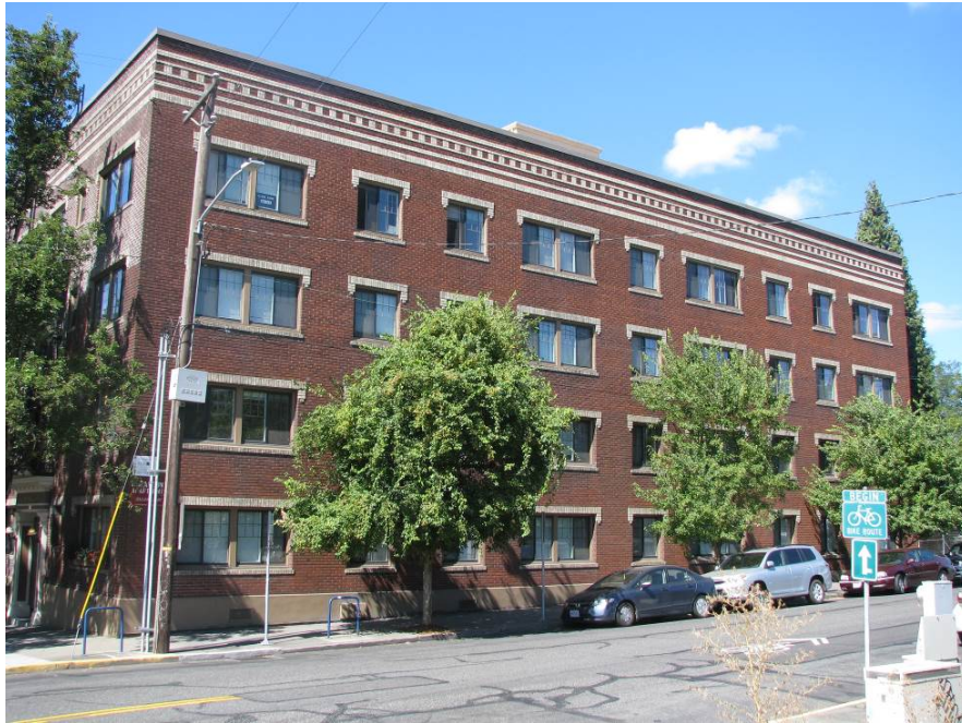
Paramount Apartments viewing northwest
