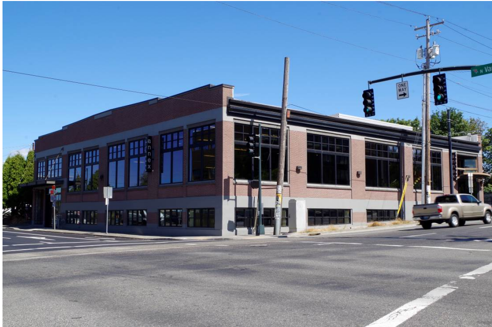
The Leftbank Annex viewing northeast
