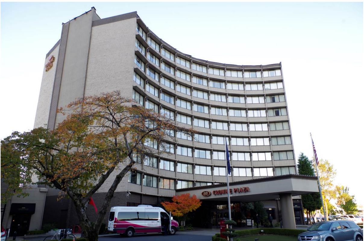
View: East elevation, viewing northwest
