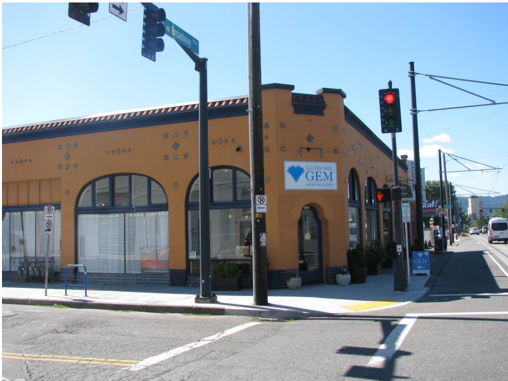
View: Secondary entrance, viewing southwest
