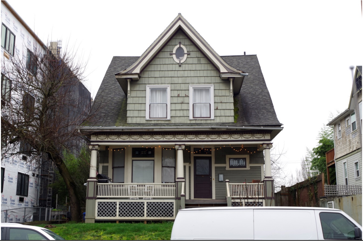
View: East façade, viewing west
