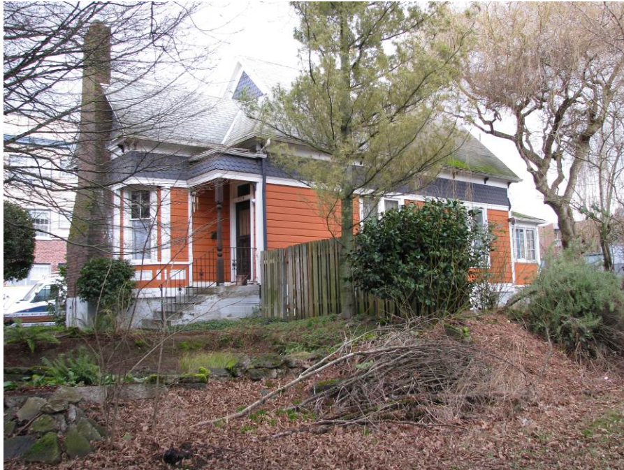
Perry and Della Coleman House viewing northeast
