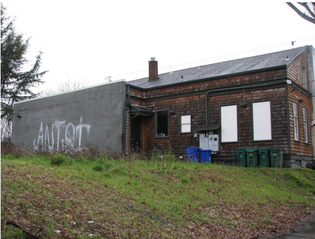
View: South elevation, viewing northwest
