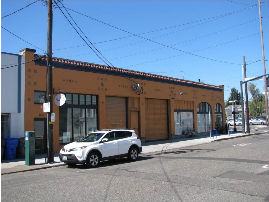
View: East elevation, viewing northwest
