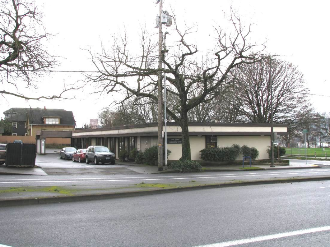
View: East and north elevations, viewing southwest
