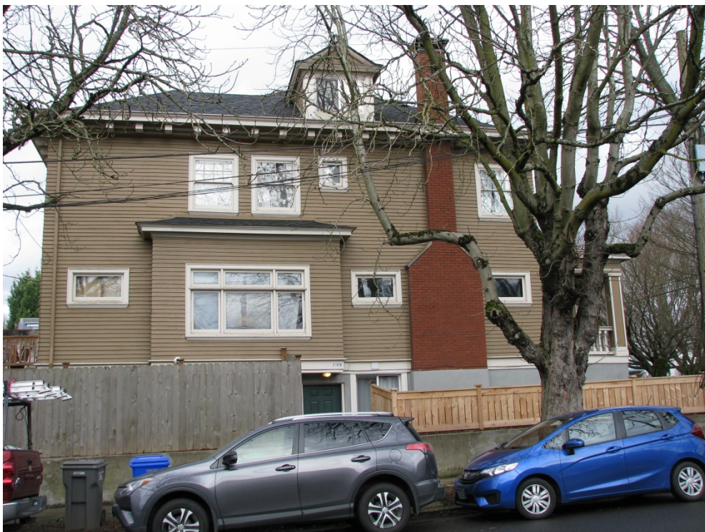
View: South elevation, viewing north
