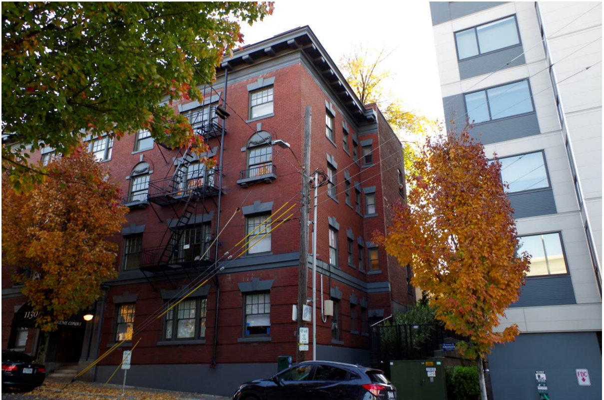
View: South elevation, viewing northeast
