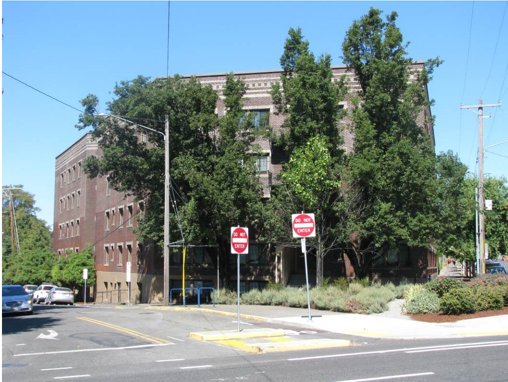
View: Façade, viewing northwest
