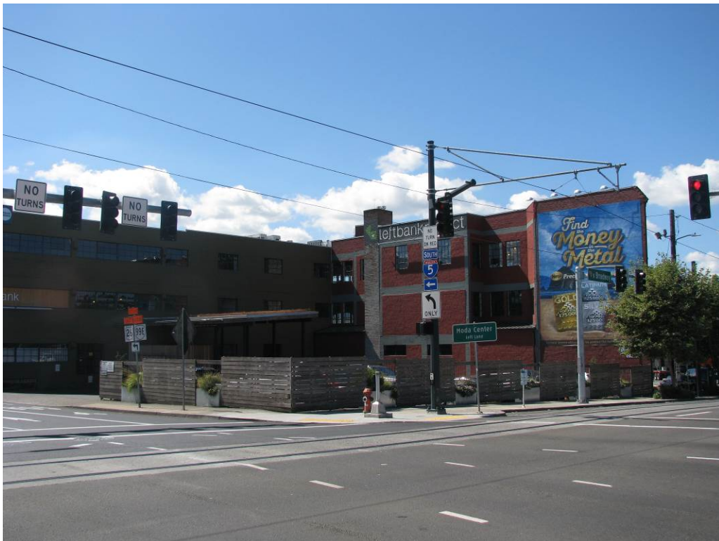
View: East elevation, viewing southwest
