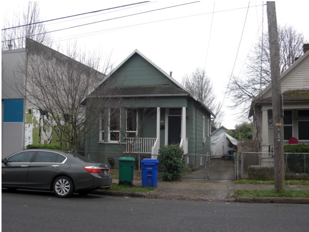
View: 226 N Page Street, North (façade) and West elevations, viewing south-southeast
