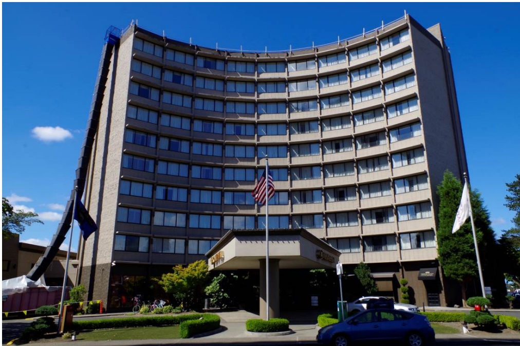
TravelLodge at the Coliseum viewing west
