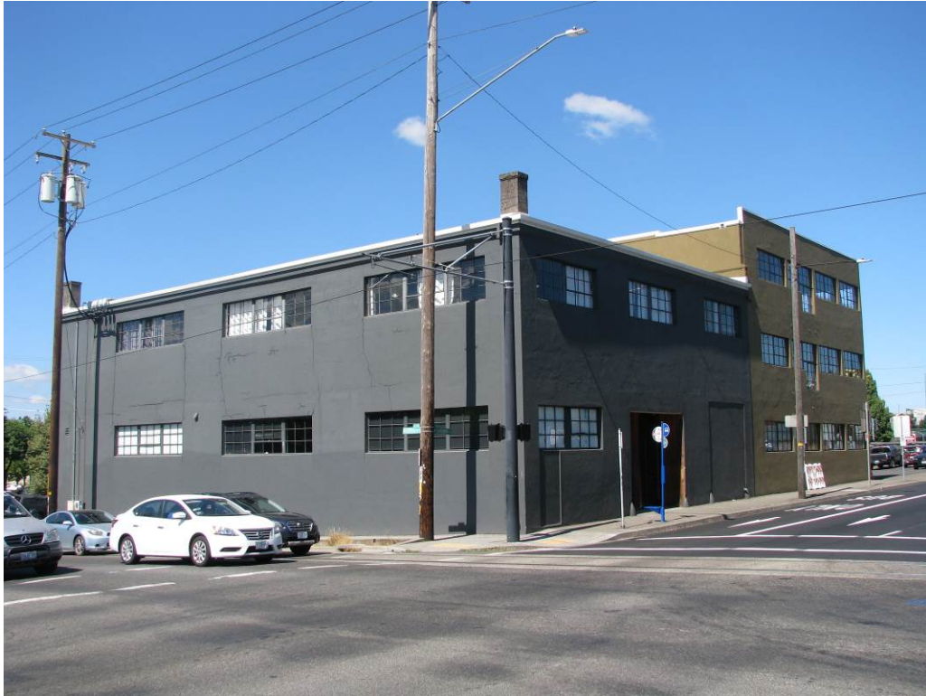
View: East and south elevations, viewing northwest
