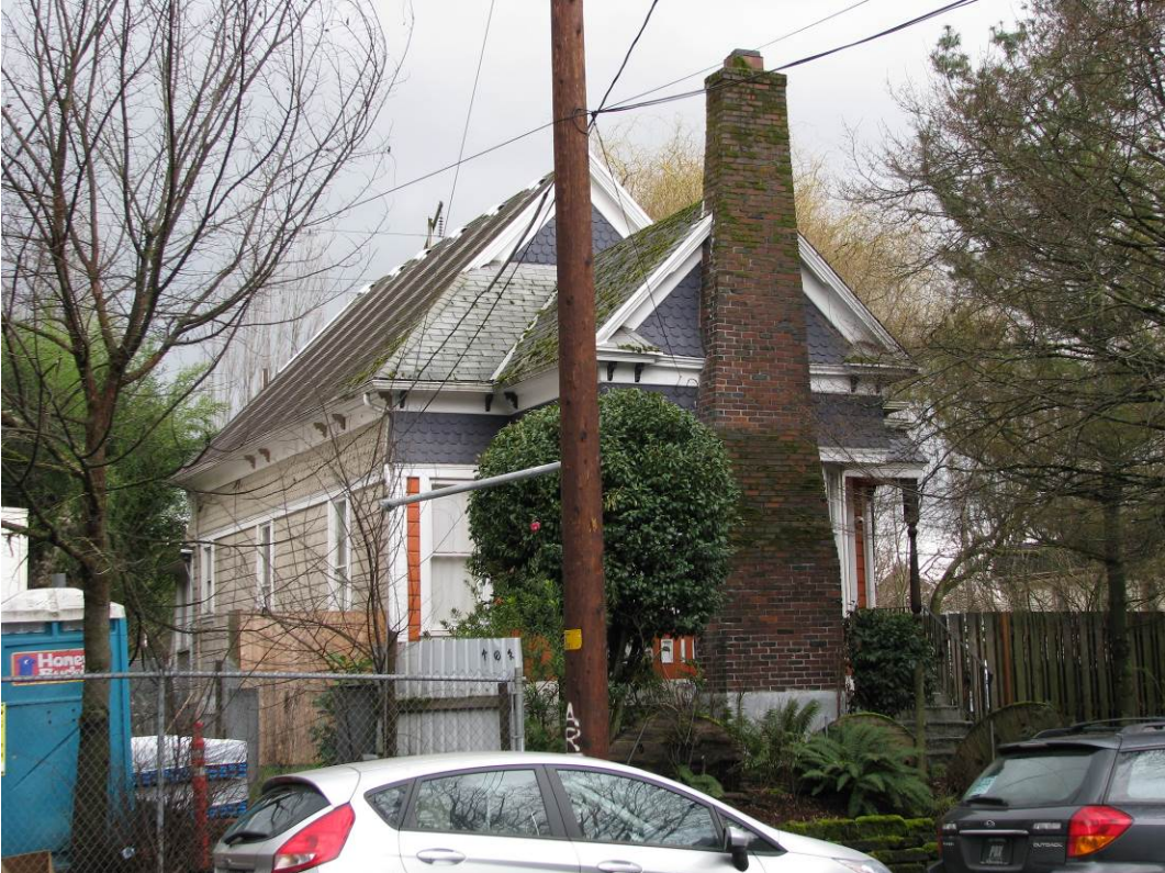
View: West and north elevations, viewing southeast
