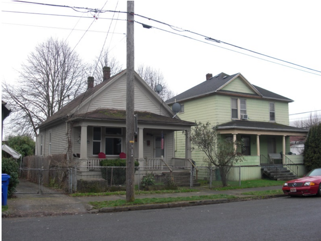
View: 230 N Page Street (left), North (façade) and East elevations, viewing south-southwest
