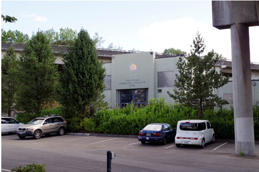
Sullivan Pumping Station viewing northeast
