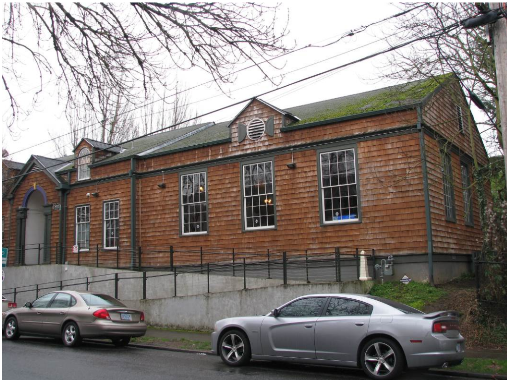
View: North façade, viewing southeast
