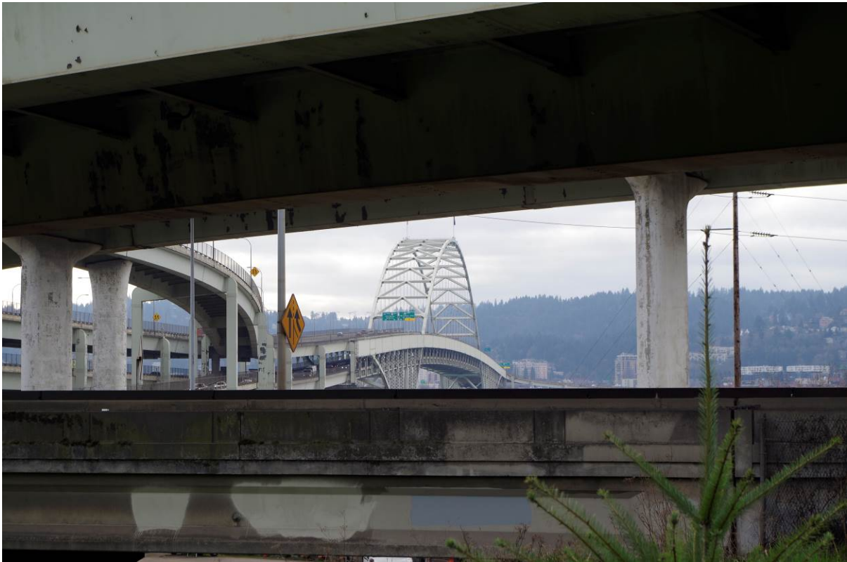
View: Fremont Bridge, viewing southwest
