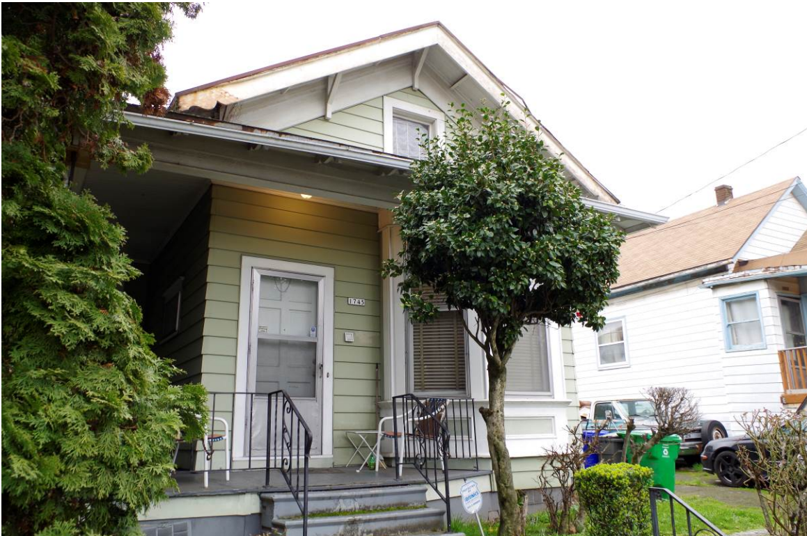
View: 1745 NE 1st Avenue, East façade, viewing northwest
