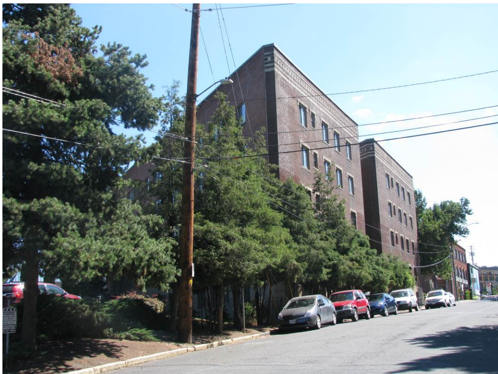
View: Southwest elevation, viewing east
