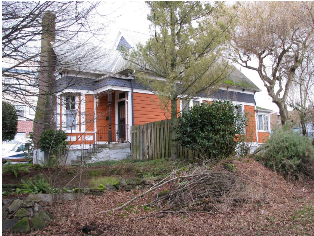
View: South elevation, viewing northeast
