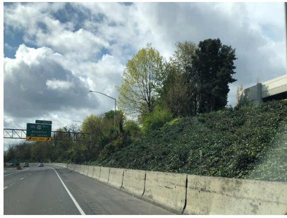
Area D, southbound I-5 with steep shoulder fill embankment, facing south.
