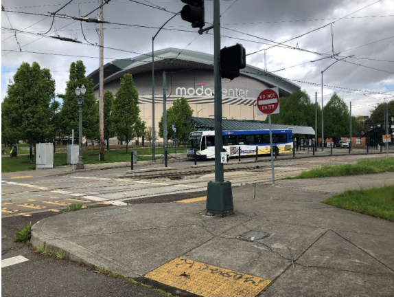
Area A, Rose Quarter Transit Center, facing northwest
