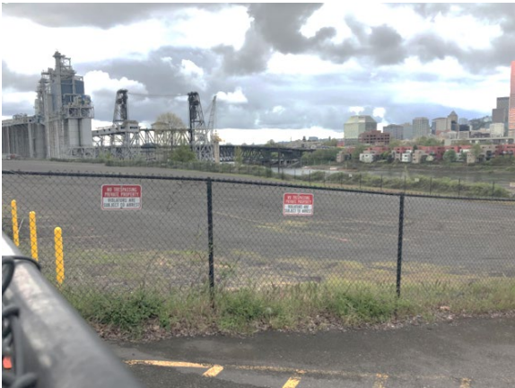
Area B, proposed contractor parking lot at the North Aegean Parking Lot, facing southwest
