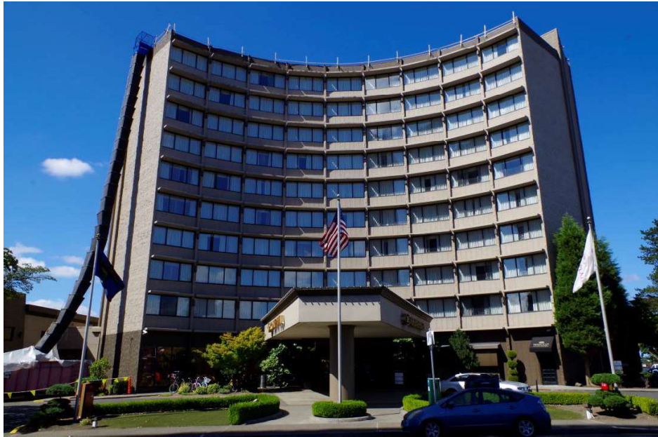
Looking west at the Travelodge at the Coliseum.
