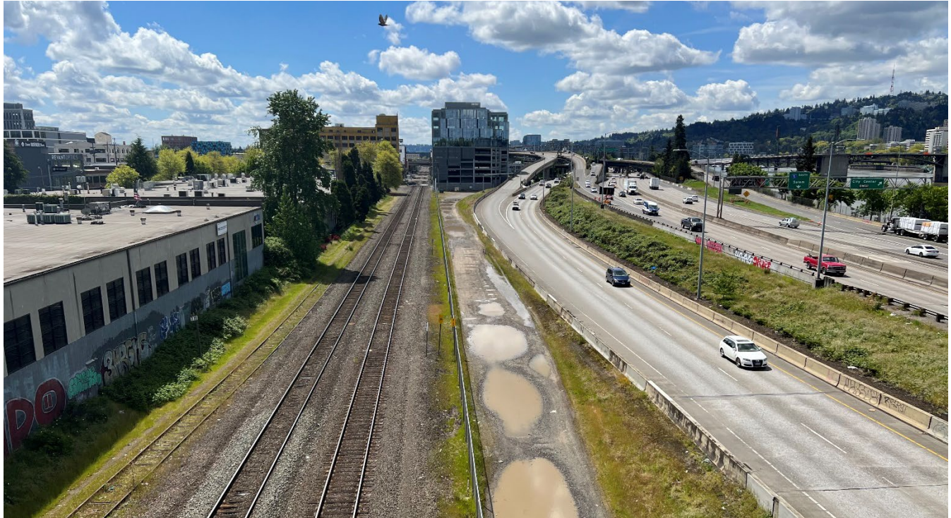
Figure 3. O&C segment, along I-5; view south from Burnside Bridge (AECOM 2022).
