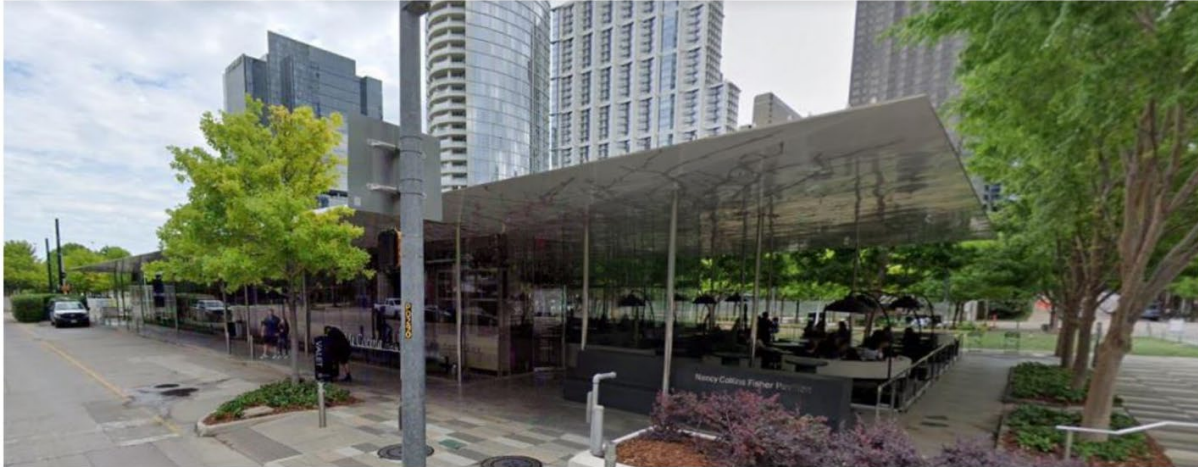
Example of light framed structure on a Cover – Klyde Warren Park
