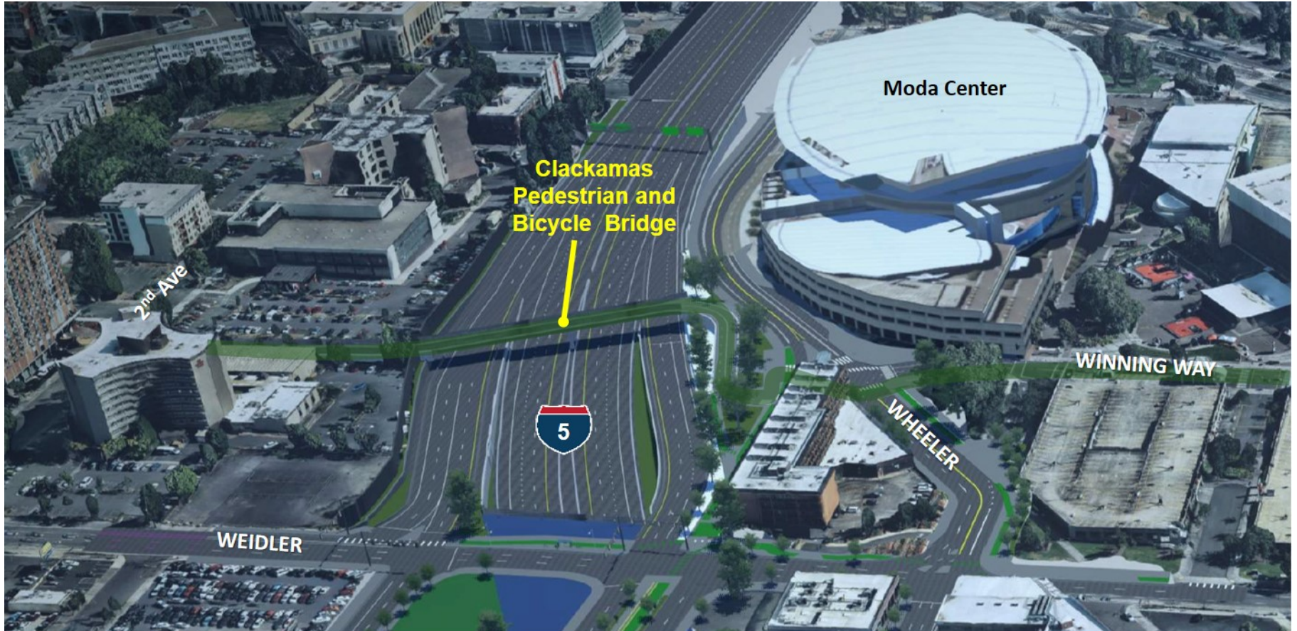
View looking south towards Moda Center
