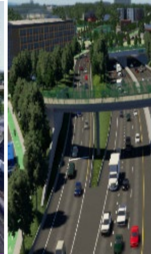
Highway Transition Zone Treatments
