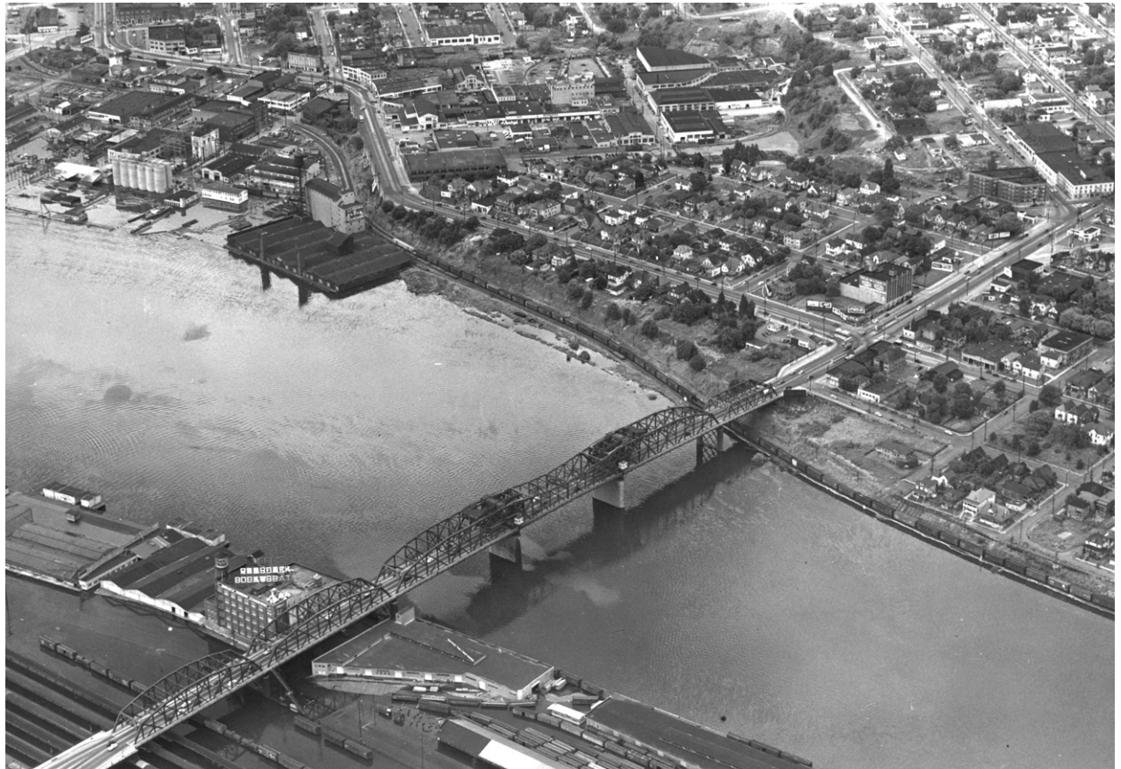
Figure 12. Western Portion of Area of Potential Impact in 1948
