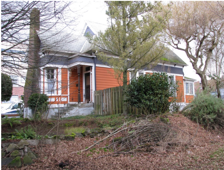
Figure 39. The Perry and Della Coleman House, looking northeast.
