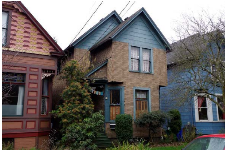
Figure 53. 72 NE San Rafael Street, looking southwest.
