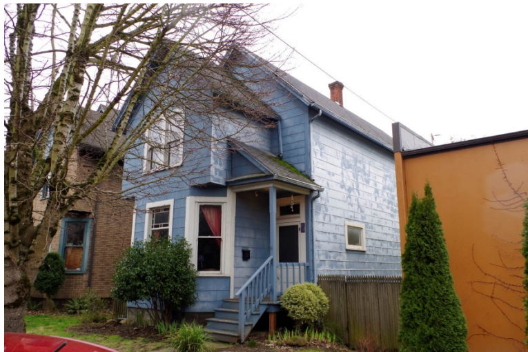
Figure 58. 66 NE San Rafael Street, looking southeast.
