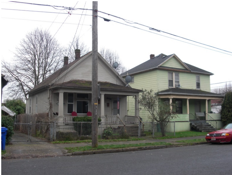
Figure 49. 230 N Page Street, looking southwest.
