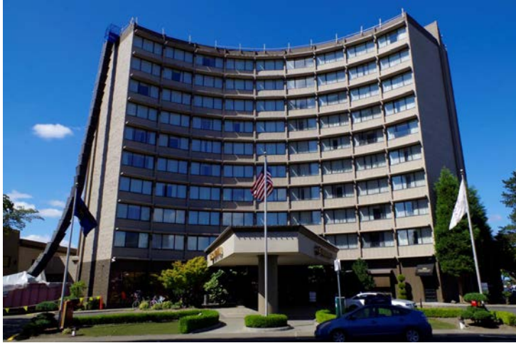
Figure 25. The Travelodge at the Coliseum, looking west.
