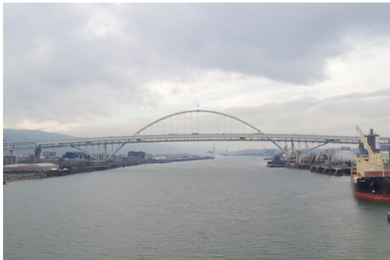
Figure 40. The Fremont Bridge, looking north.
