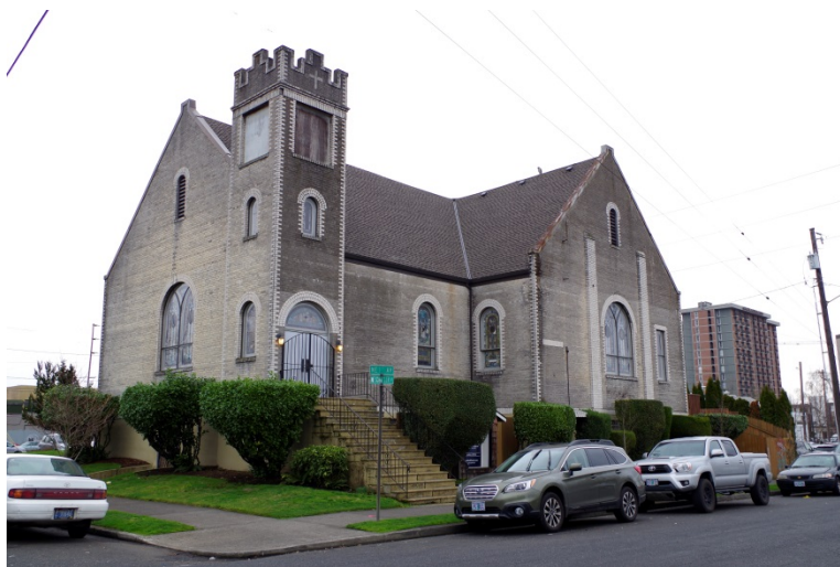
Figure 27. Mt. Olivet Baptist Church, looking southwest.
