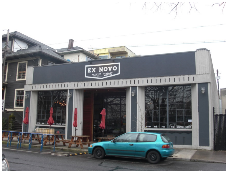
Figure 42. The Contractors' Warehouse, looking east.
