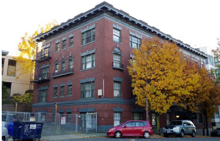
Figure 31. The Serene Court Apartments, looking southeast.
