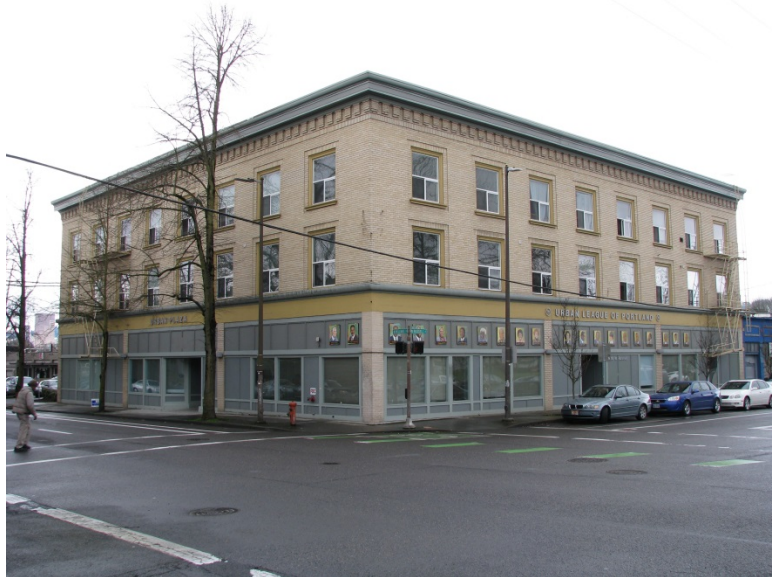
Figure 34. The Urban League of Portland, looking southwest.
