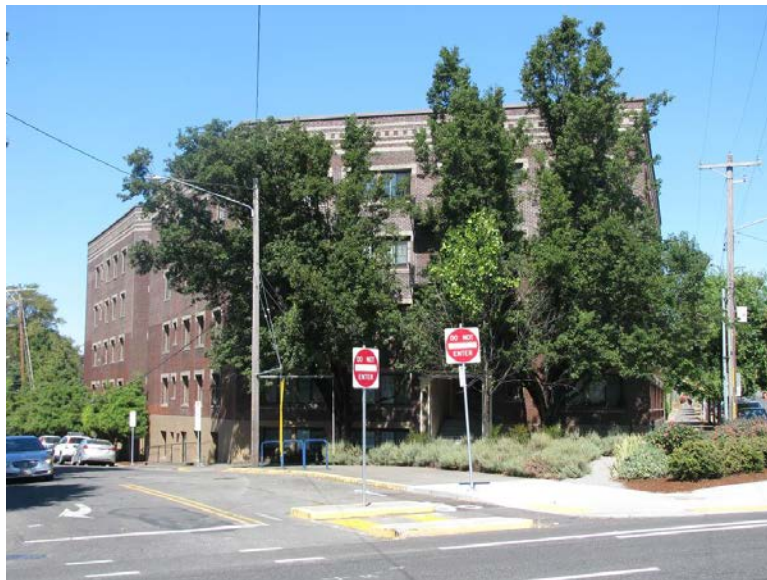
Figure 30. The Paramount Apartments, looking north.
