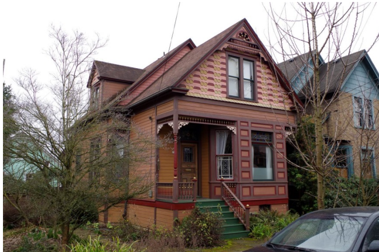
Figure 54. 76 NE San Rafael Street, looking southwest.
