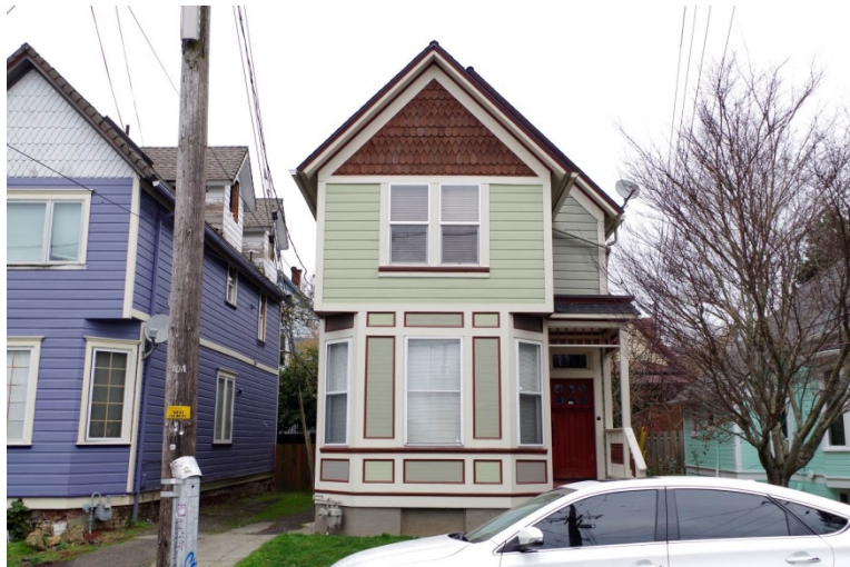
Figure 55. 73 NE Hancock Street, looking north.
