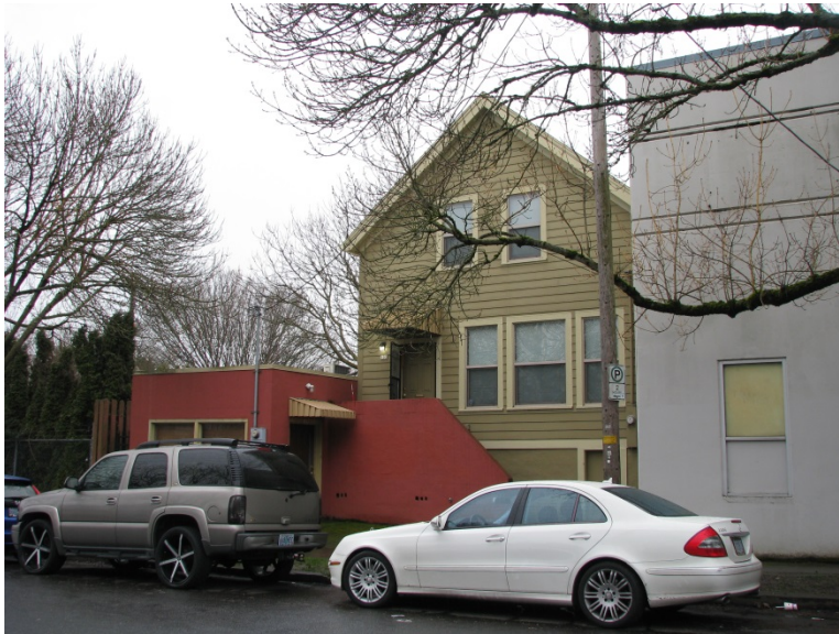
Figure 41. The John and Matilda Buckley House and Tillamook Street Barber Shop, looking north.
