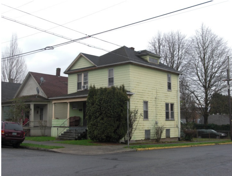
Figure 50. 236 N Page Street, looking southeast.
