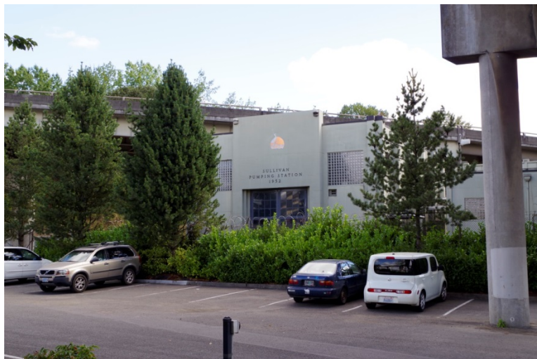
Figure 28. The Sullivan Pumping Station, looking northwest.
