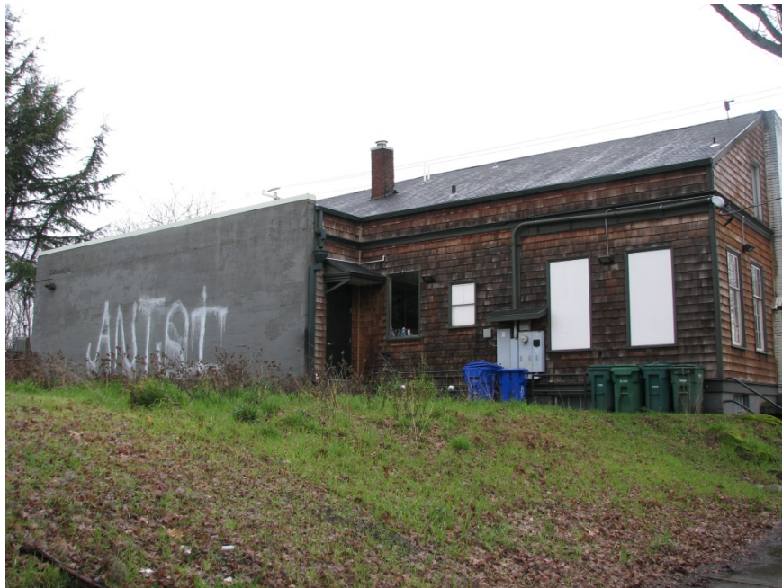
Photograph 2. Billy Webb Elks Lodge south elevation, looking northwest
