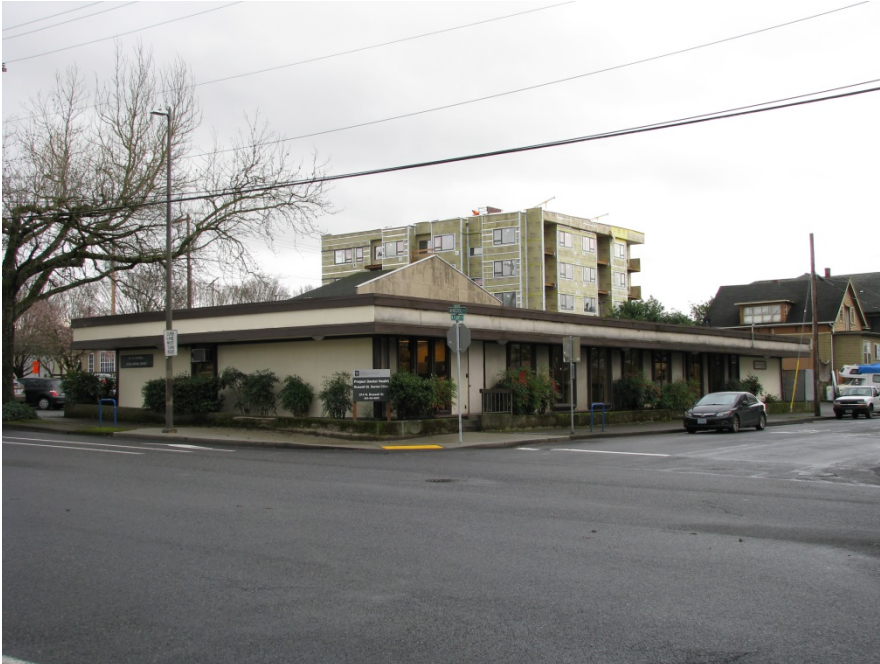
Photograph 2. The Malcom X Dental clinic west elevation, looking southeast
