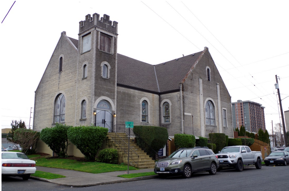
Photograph 1. Mount Olivet Baptist Church west facade, looking southeast
