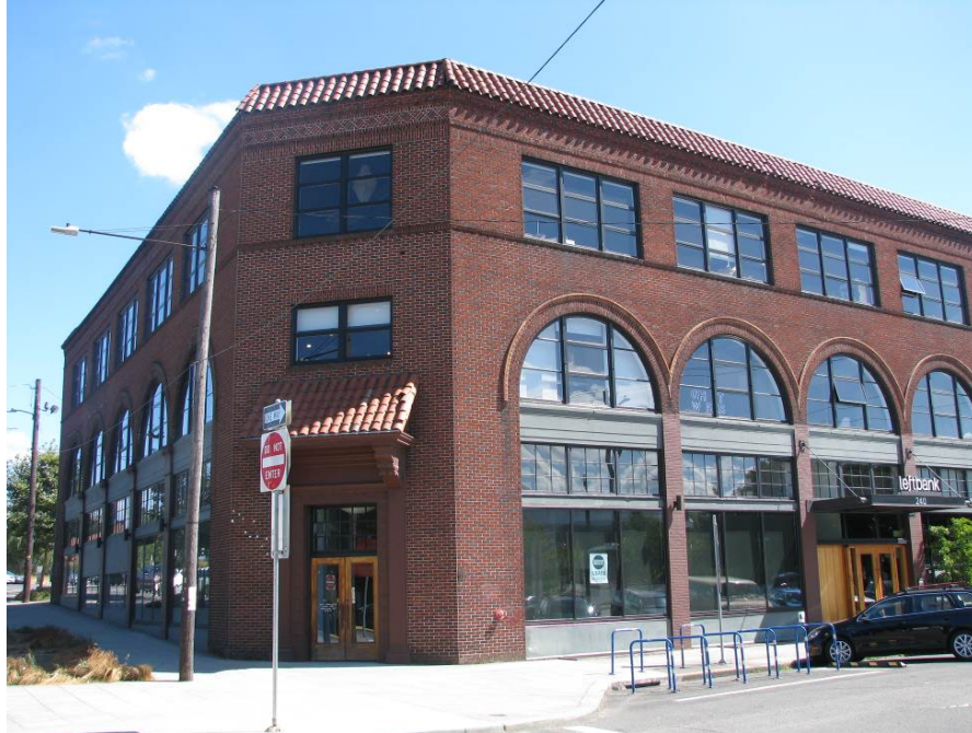
Photograph 1. The Hazelwood west facade, looking northeast
