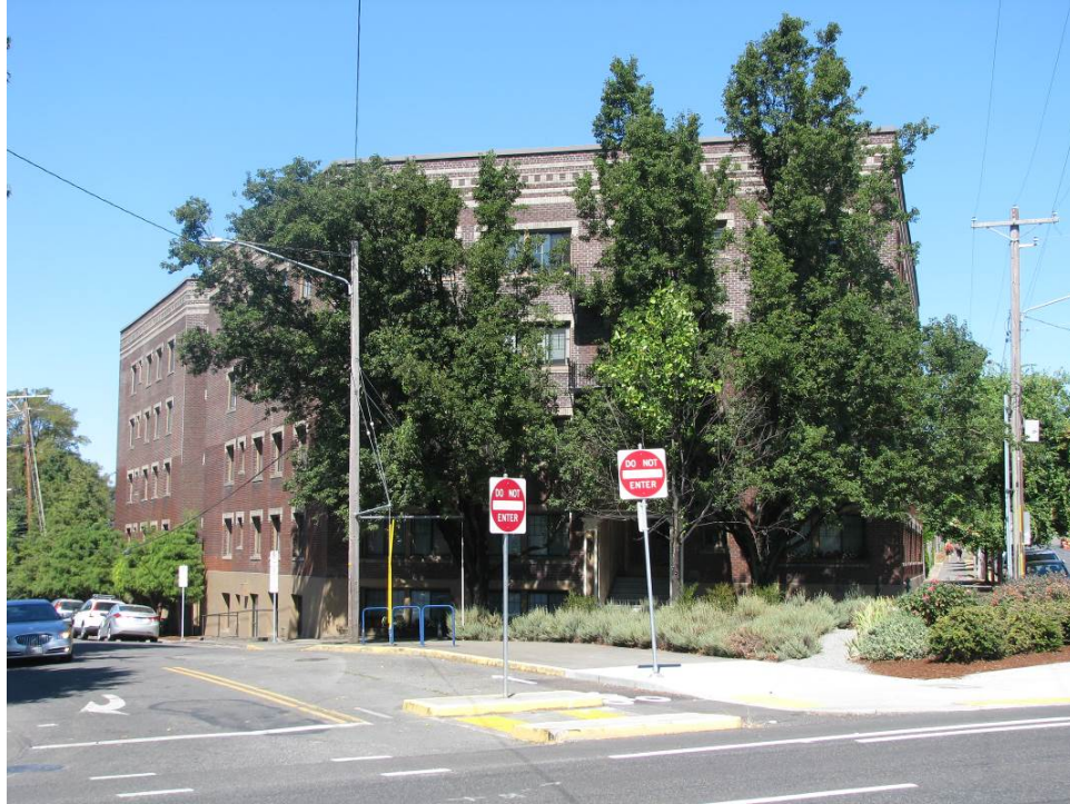
Photograph 2. The Paramount Apartments north elevation, looking southeast
