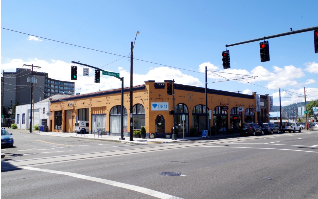
Photograph 1. W.E. Field Tile Co. Building, looking southwest
