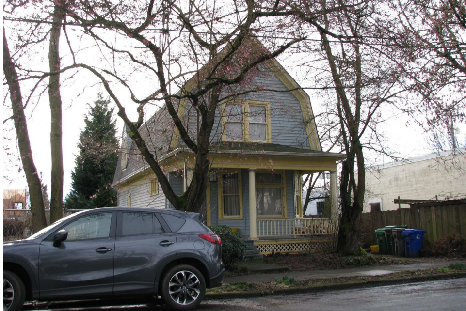
View: 20 NE Thompson Street, facing southwest
