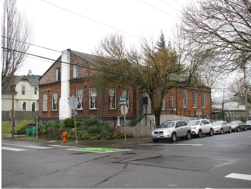
Photograph 1. Billy Webb Elks Lodge north facade, looking southwest
