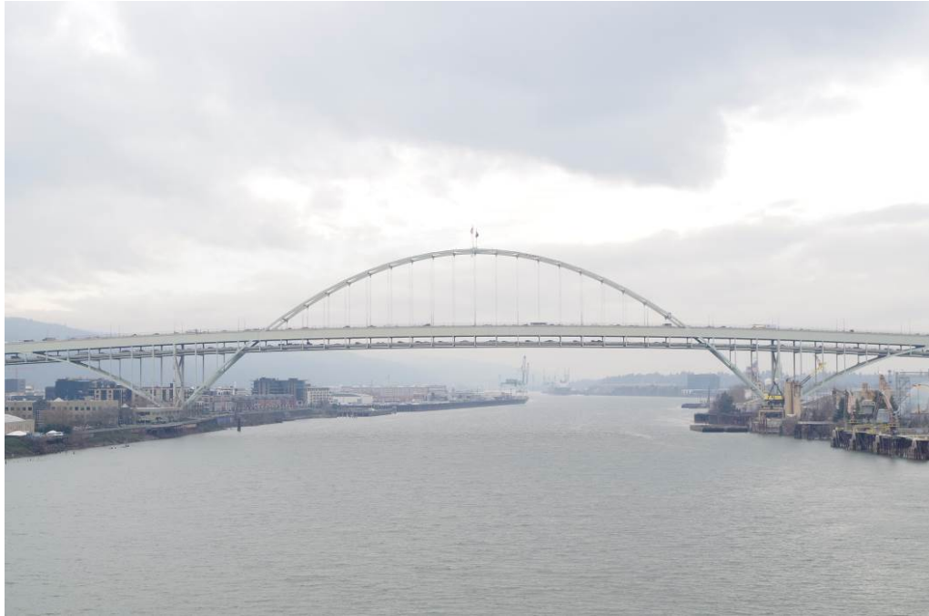
Photograph 1. Fremont Bridge, looking northwest
