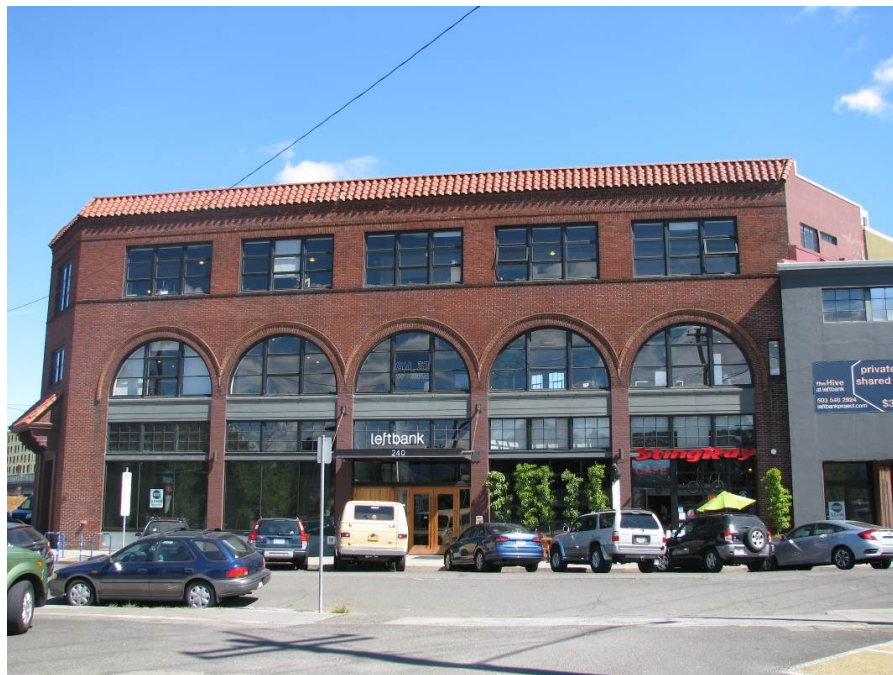
Photograph 2. The Hazelwood southwest elevation, looking northeast
