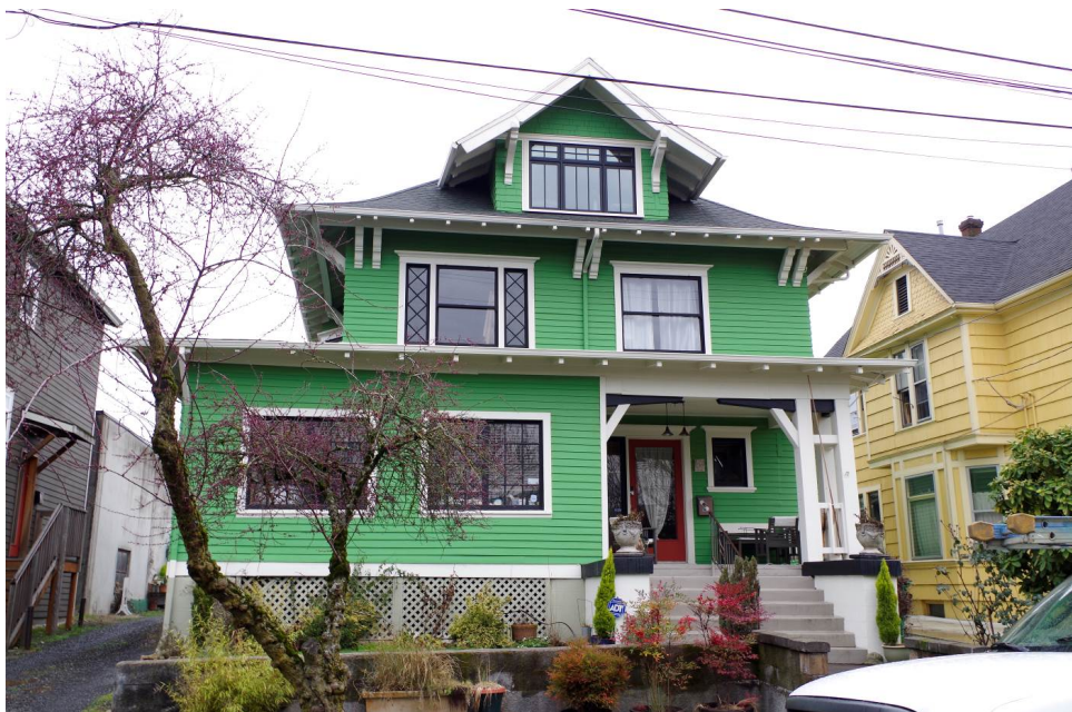
View: 23 NE San Rafael Street, facing north
