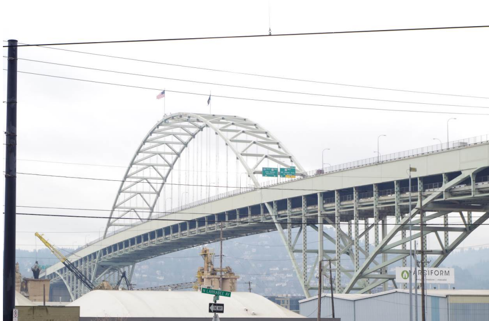
Photograph 2. Fremont Bridge, looking west
