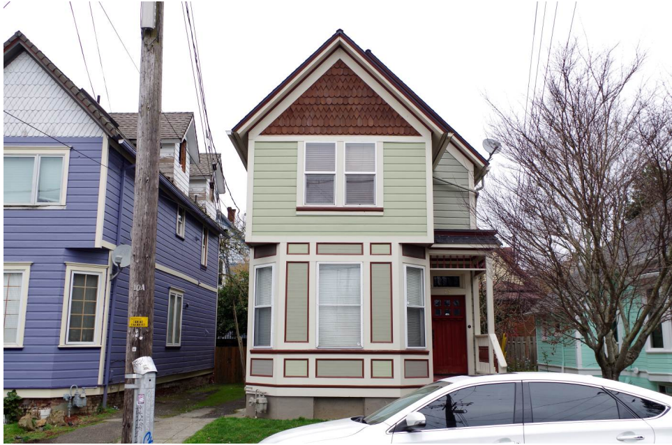
View: 73 NE Hancock Street, facing north
