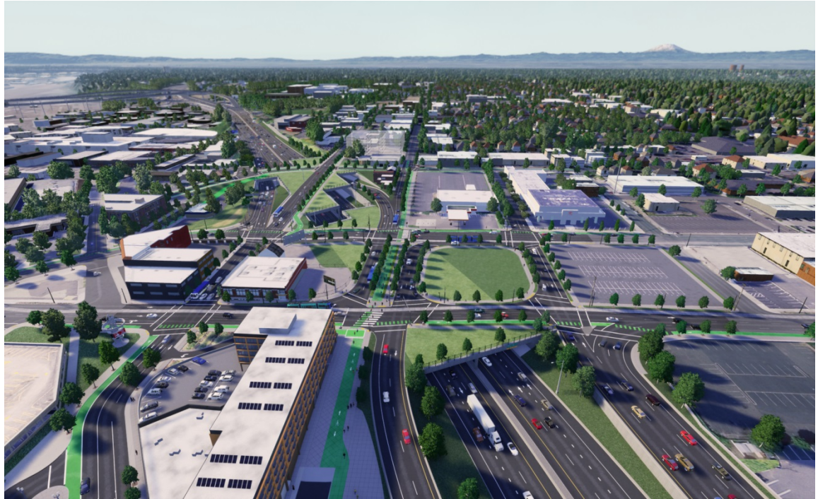
Figure 5. Broadway/Weidler/Williams and Vancouver/Hancock Highway Covers
