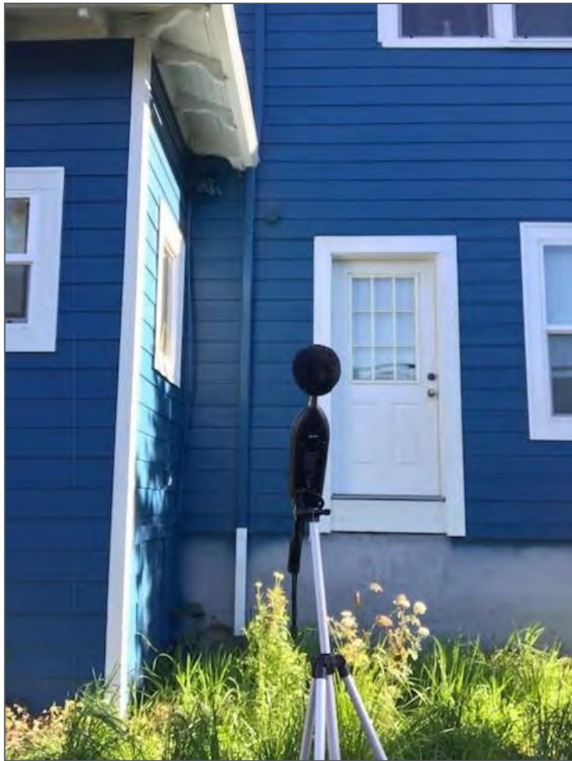
Photo 21: 2723 N Kerby Ave. (Site 6), facing east
