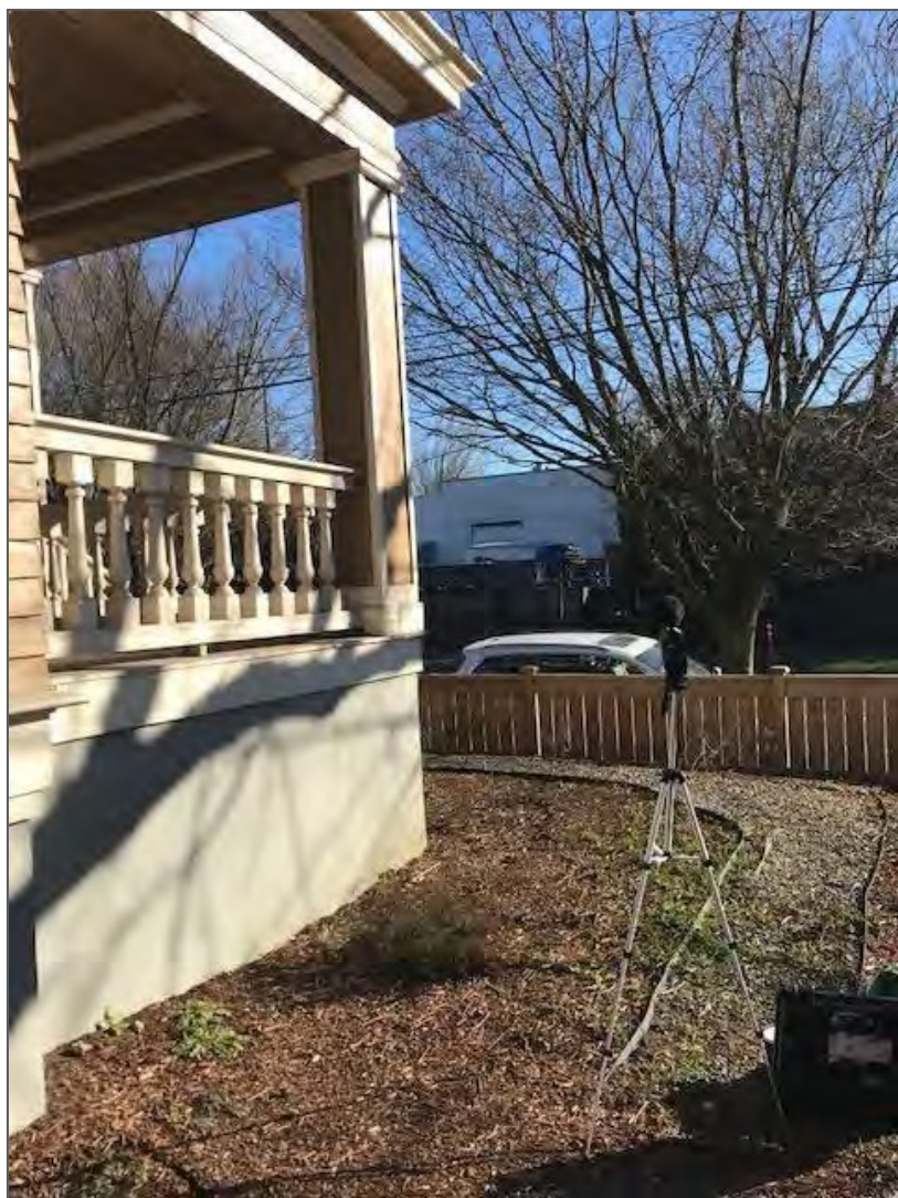
Photo 11: 2107 N Vancouver Ave. (Site 3), facing east
