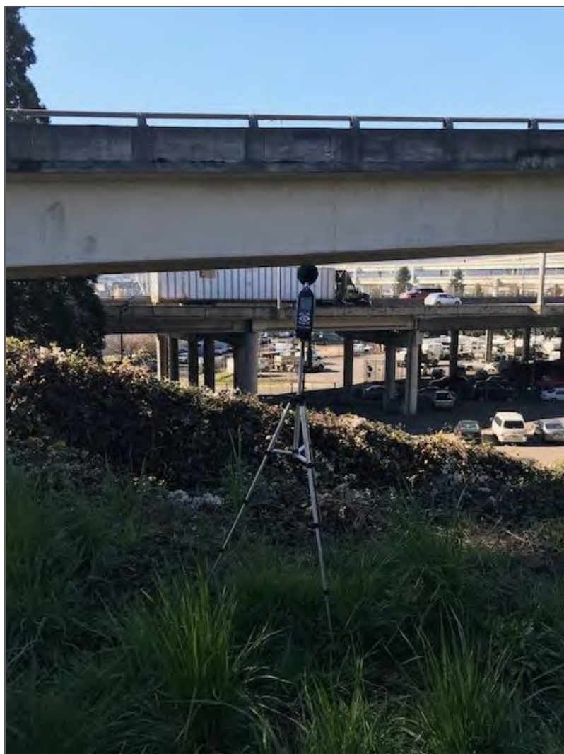
Photo 23: 2723 N Kerby Ave. (Site 6), facing west
