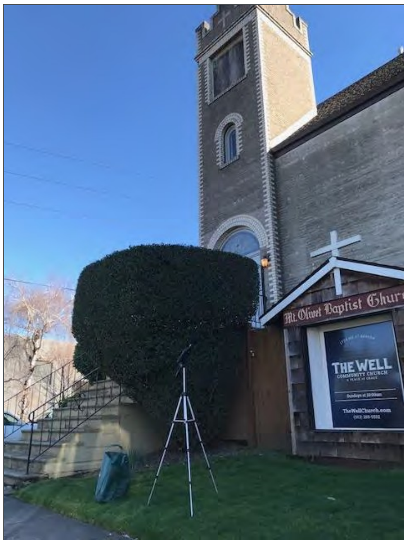
Photo 19: 1734 NE 1 st Ave. (Site 5), facing northeast
