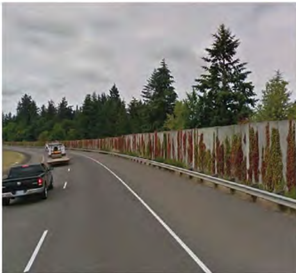
Example sound wall. Sound walls reduce noise for neighborhoods, students, and businesses
