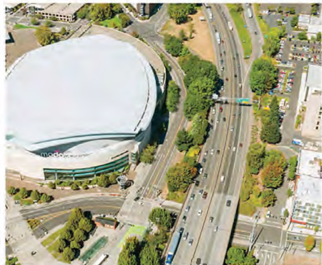
Project will maintain access to major facilities in the Project Area
