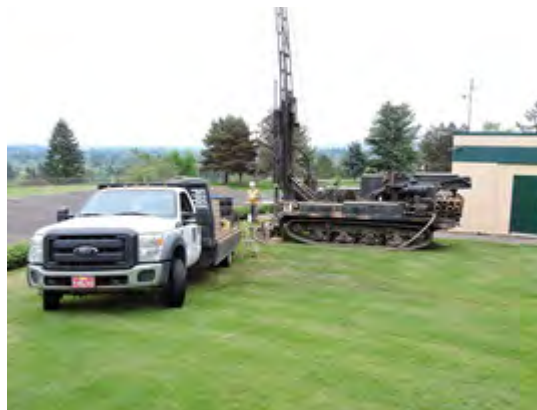
Track-mounted rig used for soil sampling on site with limited access.
