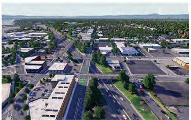
Existing overpasses over I-5
