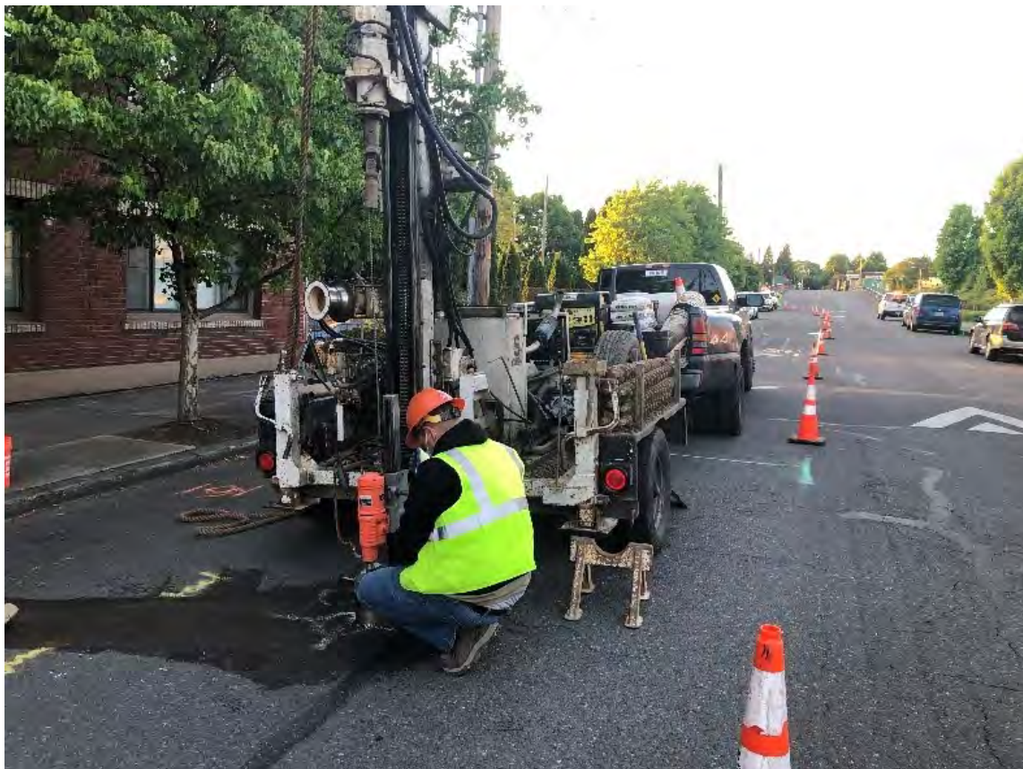
Crew in the Rose Quarter taking pavement core samples
