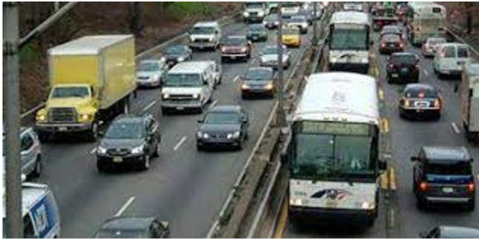
Figure 22 Managed contraflow lanes, example Route 495 North Bergen, NJ
