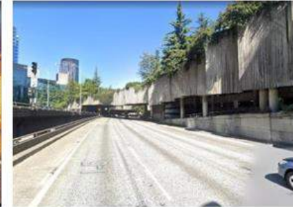
I-5 Freeway Park Seattle, WA 11' Lanes 6' Inside Shoulder 8' Outside Shoulder
