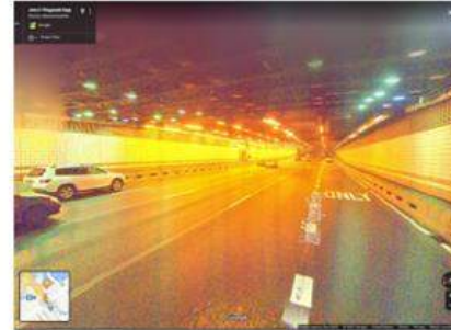
I-93 Central Artery, MA 12' Lanes 0' Inside Shoulder 0' Outside Shoulder
