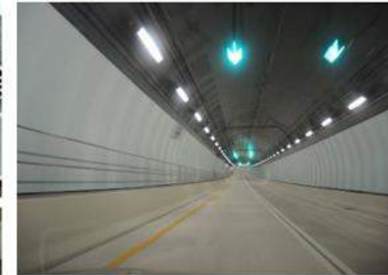
Port of Miami Tunnel, FL 12' Lanes 2' Inside Shoulder 2' Outside Shoulder
